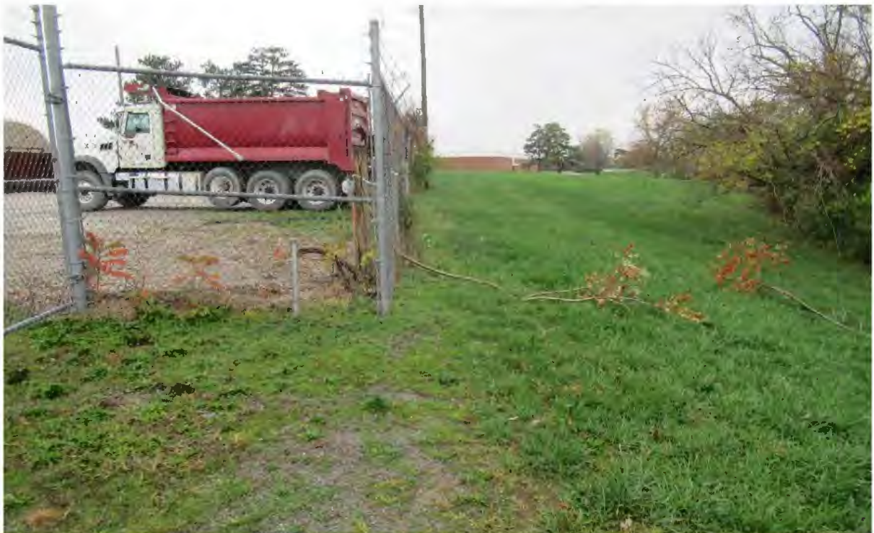
Figure 1-17: West Side of Fenced Public Works Facility
