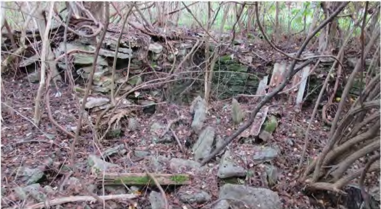
Figure 1-5: Foundation Walls at Site 15Cp81
