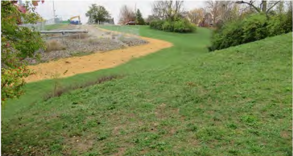
Figure 1-26: East End of Eastern Project Segment
