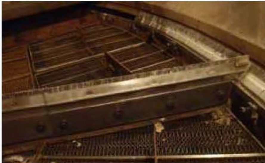
Figure 4-8 Installed Adaptive Brush Radial and Circumferential Seals (Courtesy of Sealeze® Power)
