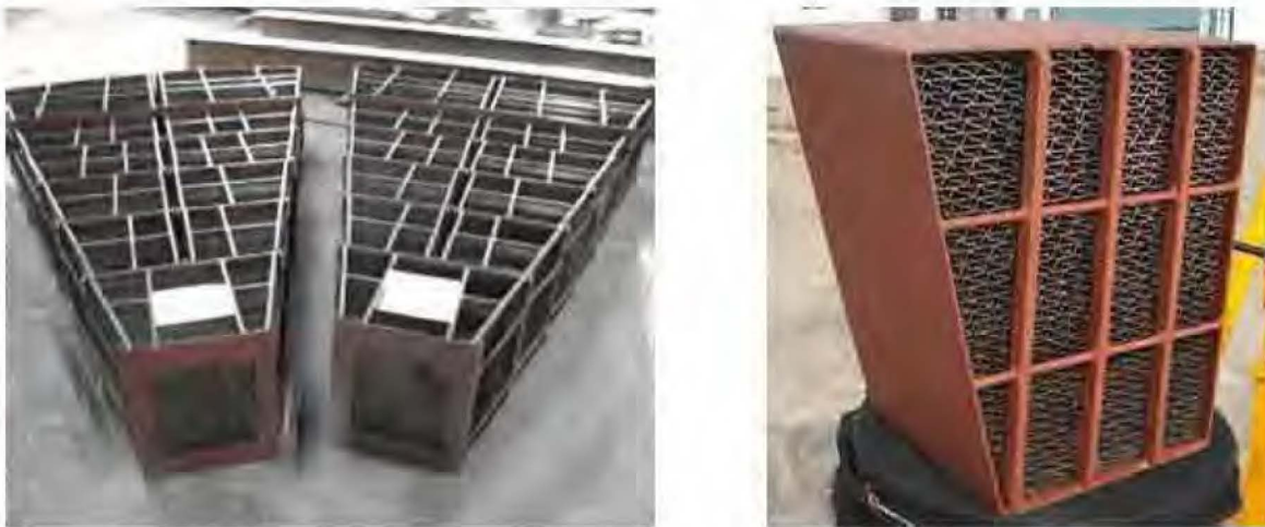
Figure 4-6 Air Preheater Replacement Rotor Frames and Basket Assemblies
