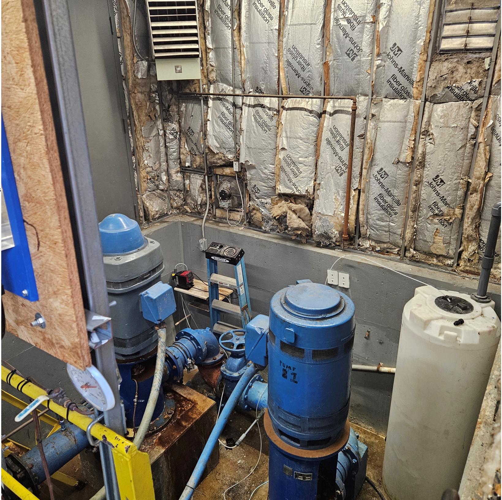
The pumps in this picture are vertical stack pumps that have had their motors rebuilt approximately 4 times each and will not run at the full capacity of 1,000 gallons per minute due to wear. Both pumps also leak. We have tried resealing them, but the pump housings are too worn to seal completely.
