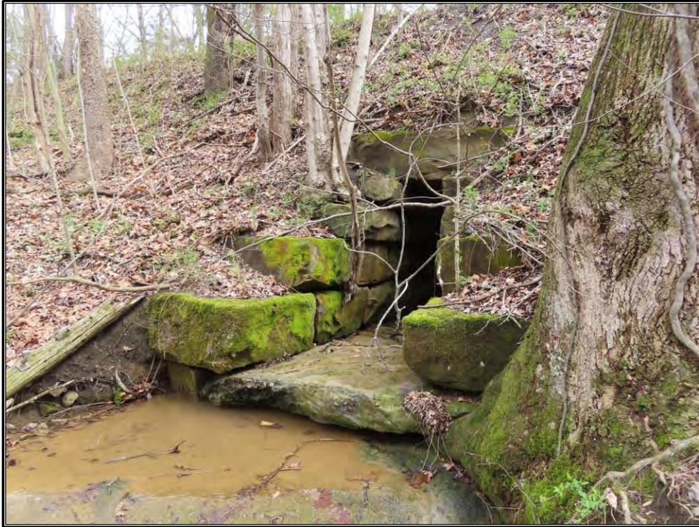
Figure 13. CRA 3: West elevation of the cut limestone railroad culvert, looking northeast.
