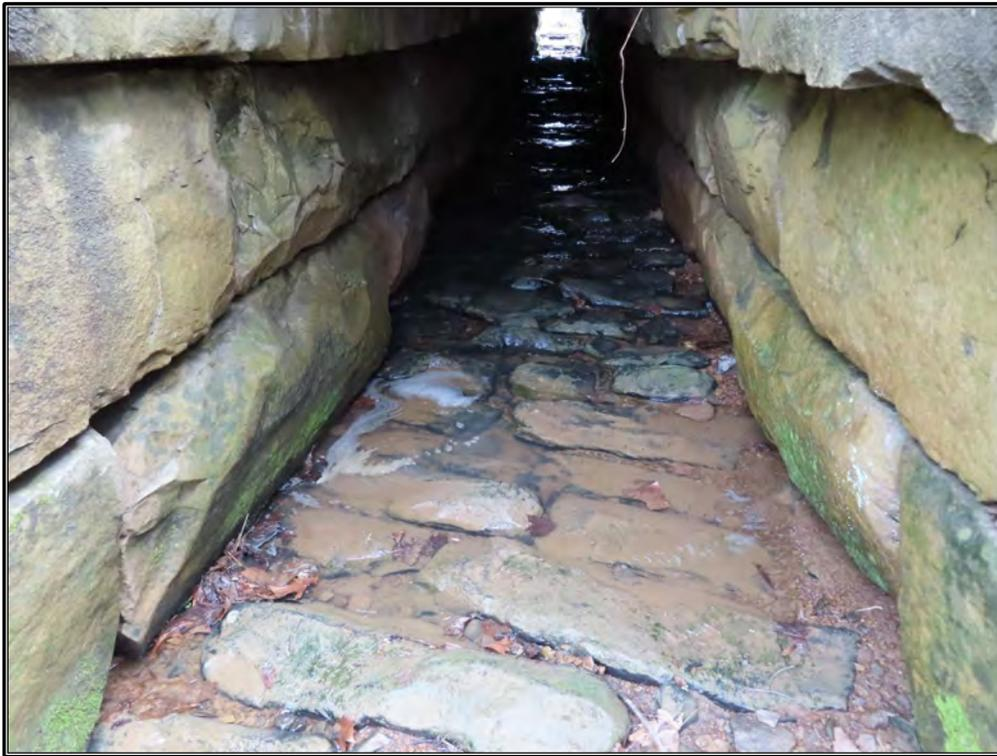
**Figure 15. CRA 3: Overview of the culvert's interior showing limestone block floor, looking east.**
