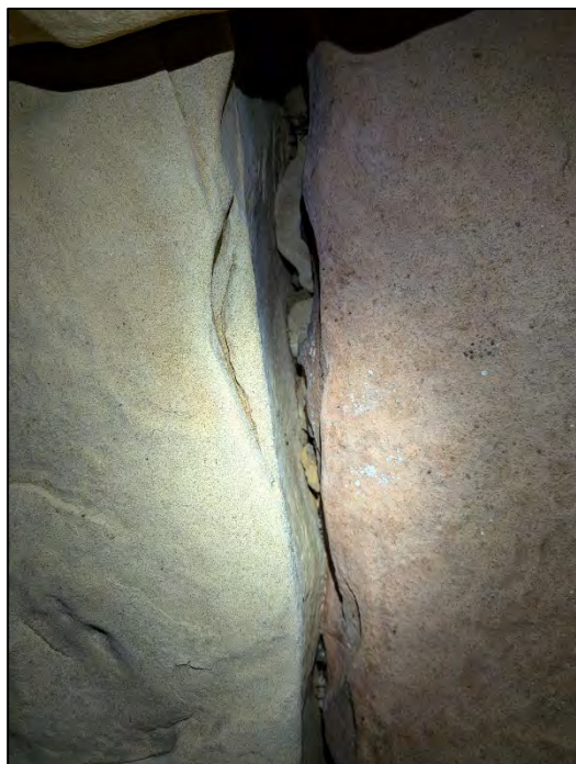
Potential bat roost location in the wall of the culvert
