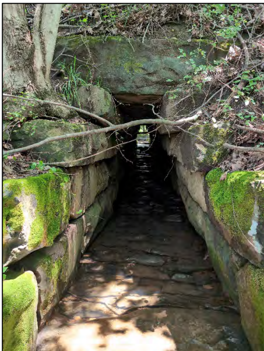
Culvert entrance showing cut stone walls and roof
