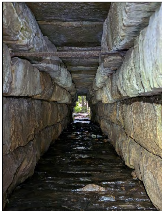
Internal passage of culvert
