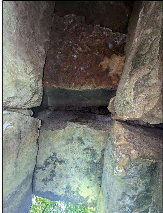
Potential bat roost location in the ceiling of the culvert
