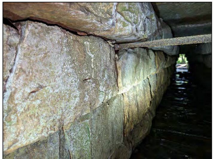
Interior wall of the culvert showing possible roost locations for bats
