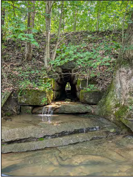
Historic railroad culvert entrance (37.098622, -86.998199)
