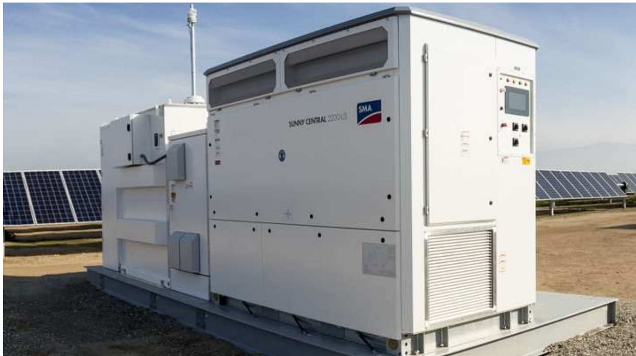
Picture (4) Industrial Solar Inverter 4
