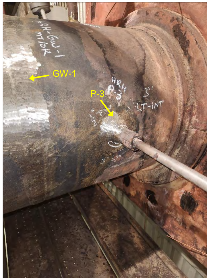
Fig. 17. Photographs of the inspection locations on the Hot Reheat piping system.
