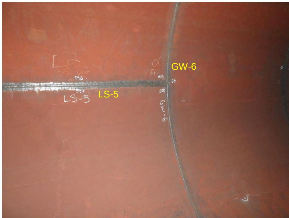
Fig. 58. Photographs of the inspection locations on the deaerator storage tank.
