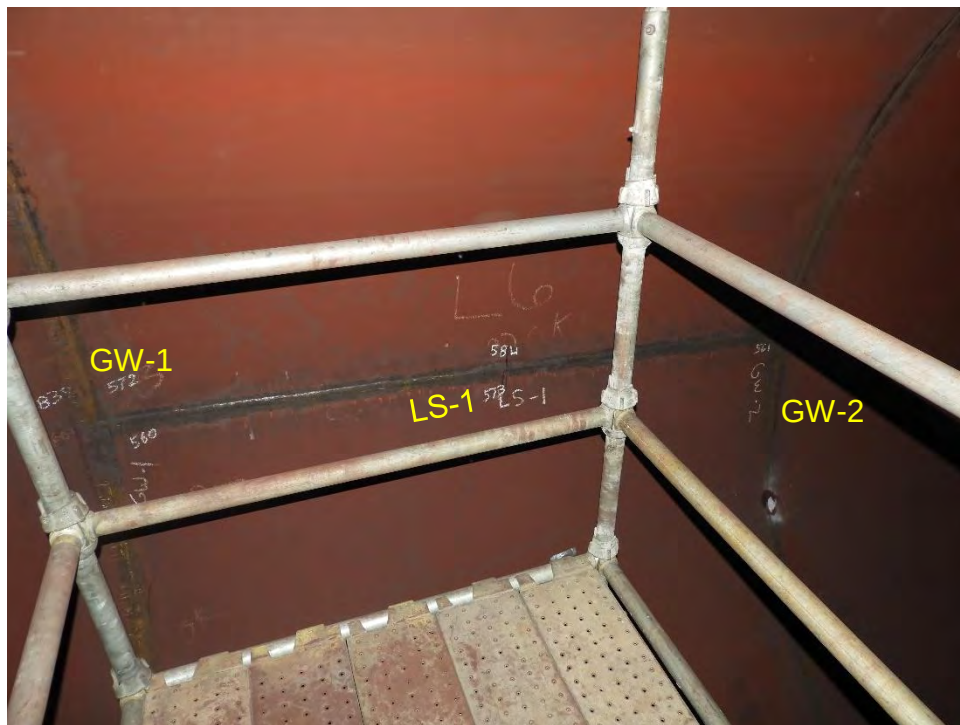
Fig. 53. Photographs of the inspection locations on the deaerator storage tank.
