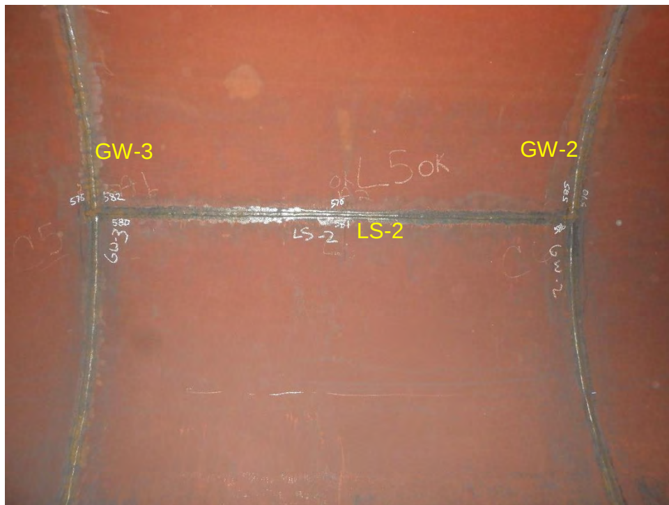
Fig. 55. Photographs of the inspection locations on the deaerator storage tank.
