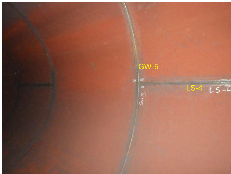
Fig. 57. Photographs of the inspection locations on the deaerator storage tank.
