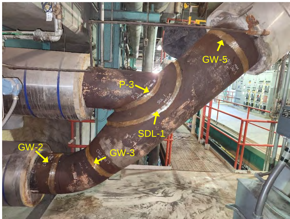
Fig. 32. Photographs of the inspection locations on the Cold Reheat piping system.
