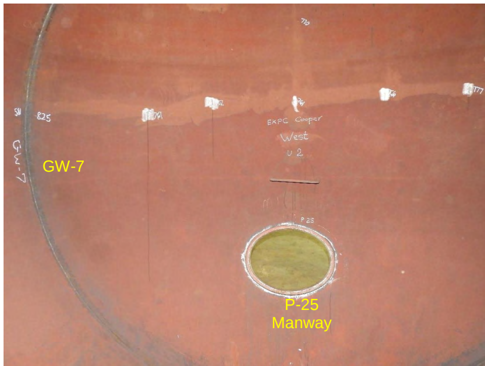
Fig. 60. Photographs of the inspection locations on the deaerator storage tank.
