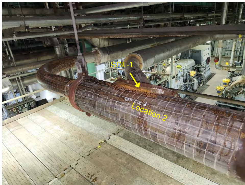
Fig. 36. Photographs of the inspection locations on the Boiler Feedwater Discharge piping system.
