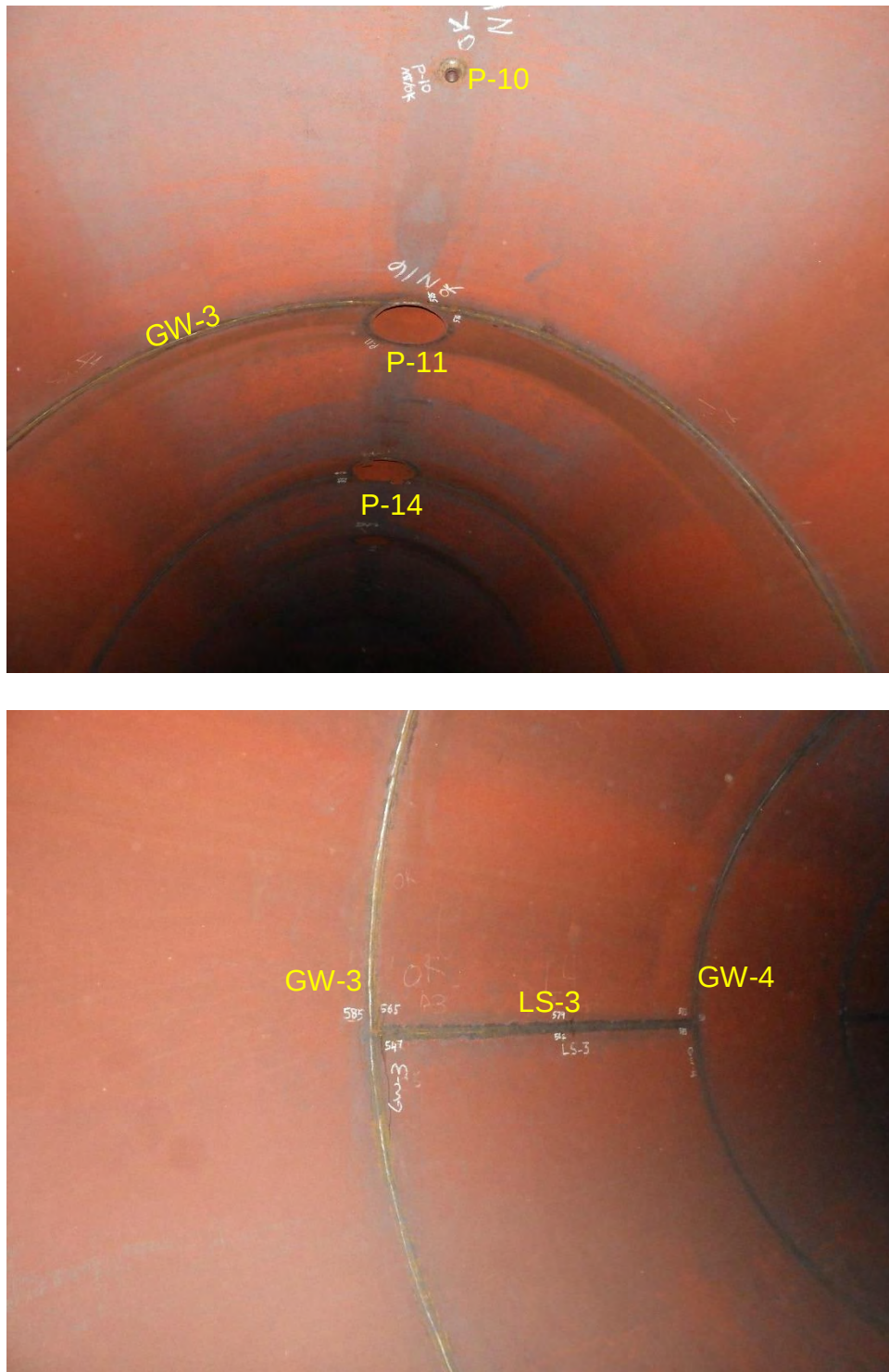
Fig. 56. Photographs of the inspection locations on the deaerator storage tank.
