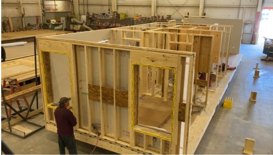
Figure A5. Bay 4 – Interior Partition Set
