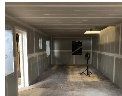
Figure 11: Drywall installed on all exterior walls and ceiling.
