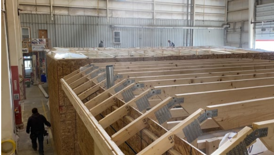
Figure A14. Bay 13 in the back - Flooring, Electrical Hookups, Interior Trim.
