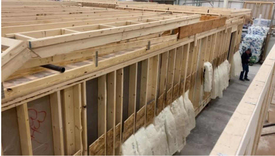
Figure A8. Bay 7 - Exterior Insulation and Drywall.
