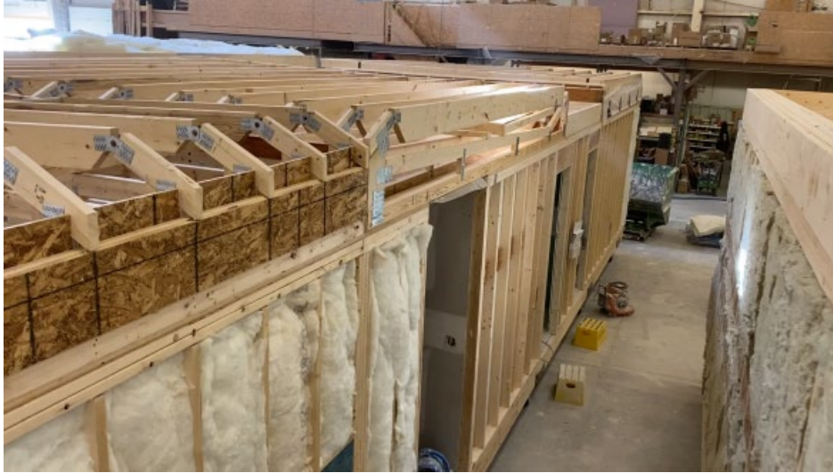
Figure A11. Bay 10 - Roof Sheathing and Exterior Wall Sheathing.
