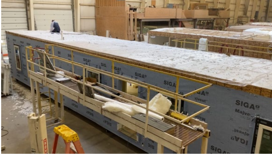
Figure A15. Bay 14 - Interior Trim, Electrical Tests, Plumbing Tests.
