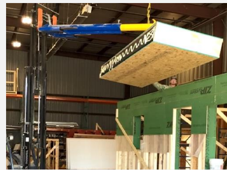
Figure 10: Crane lifting roof onto walls.
