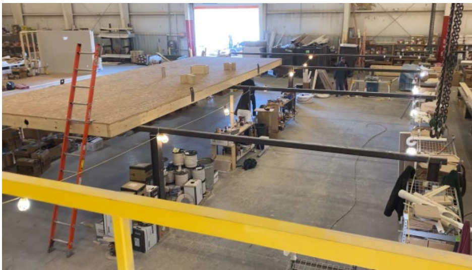
Figure A3. Bay 2 - Raised Plumbing/Electrical Jig
