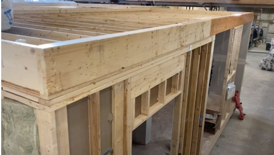
Figure A10. Bay 9 Roof Sheathing, Drywall Finish and Sanding.
