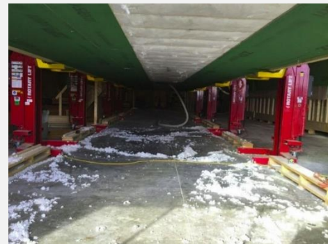
Figure 19: Insulation, and partially installed sheathing.
