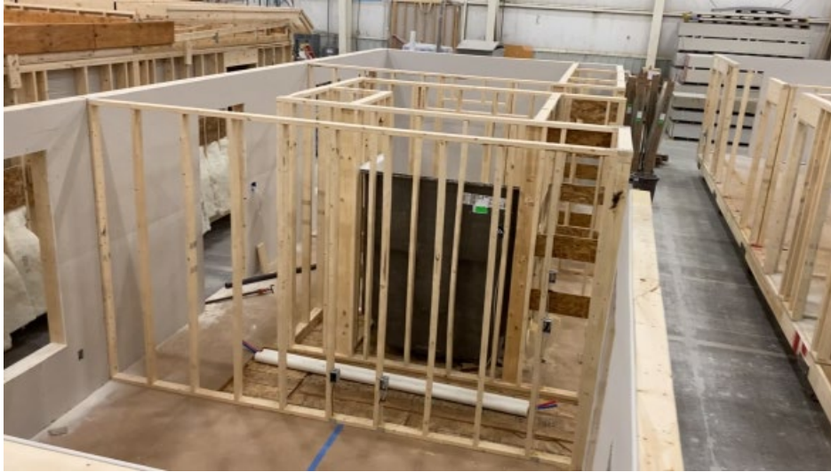
Figure A7. Bay 6 - Rough Electrical and Plumbing, Drywall, and Roof Set.
