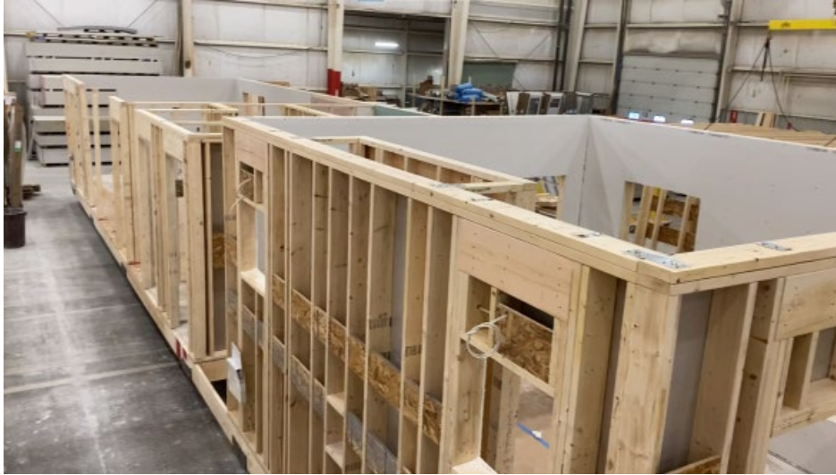
Figure A6. Bay 5 - Rough Electrical and Plumbing
