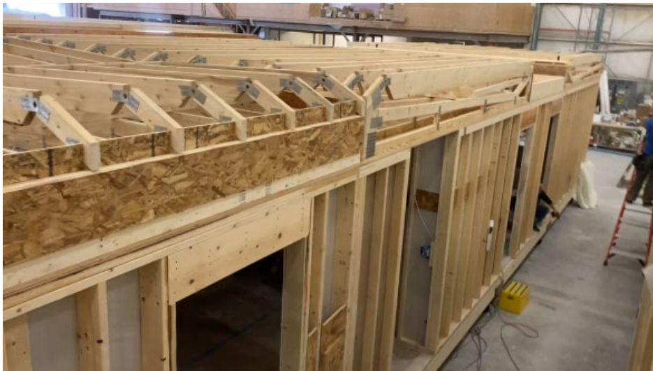
Figure A9. Bay 8 - Exterior Insulation, Drywall Finish and Sanding.
