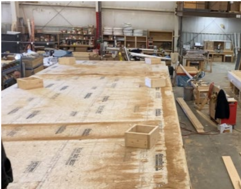
Figure A2. Bay 1 - Floor Framing and Decking
