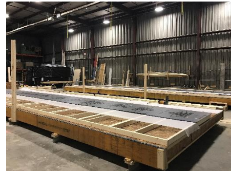
Figure 8: Exterior walls being built on deck.
