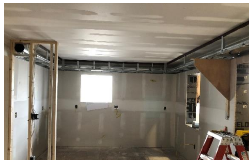
Figure 12: Installation of HVAC soffit and interior partitions.
