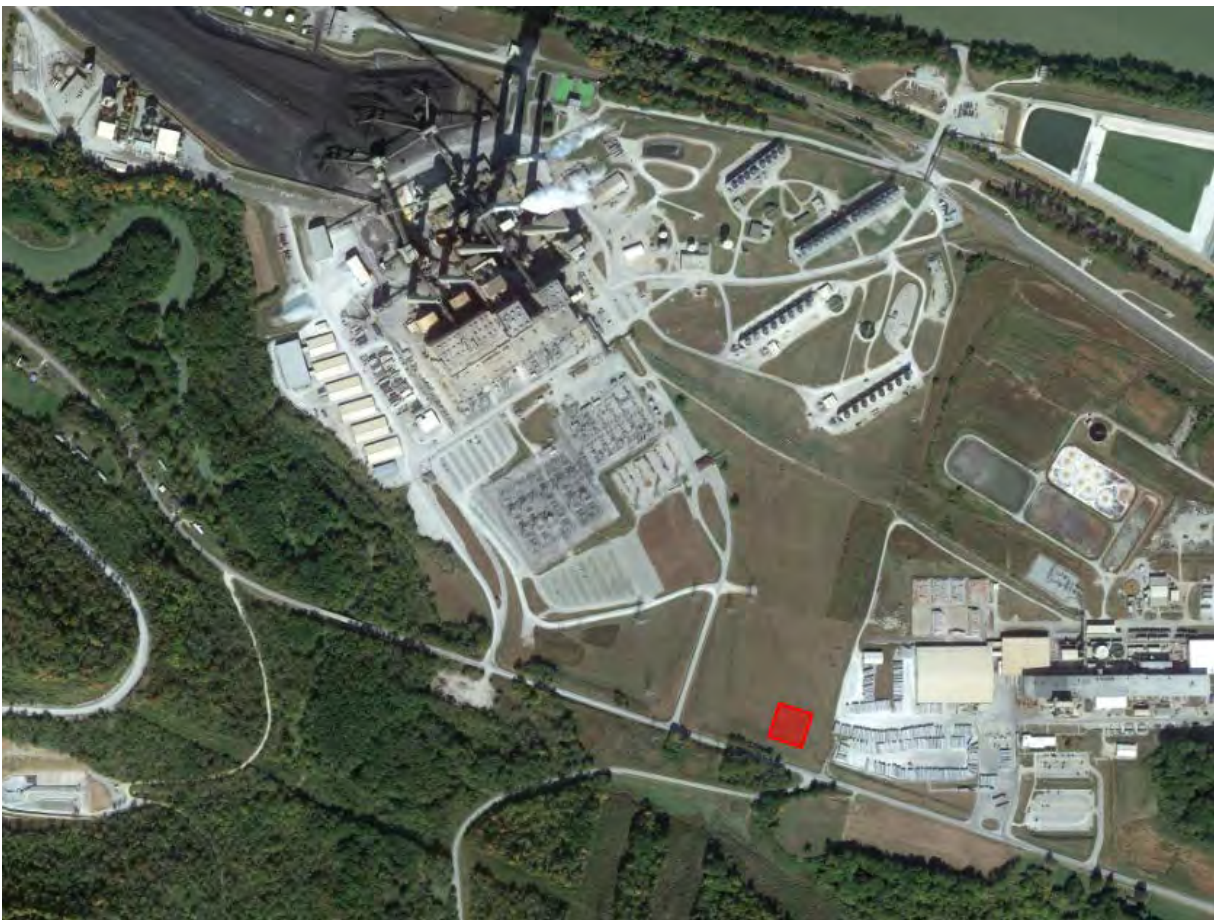
Figure 2: EKPC Spurlock Power Station with M&R Station Highlighted
