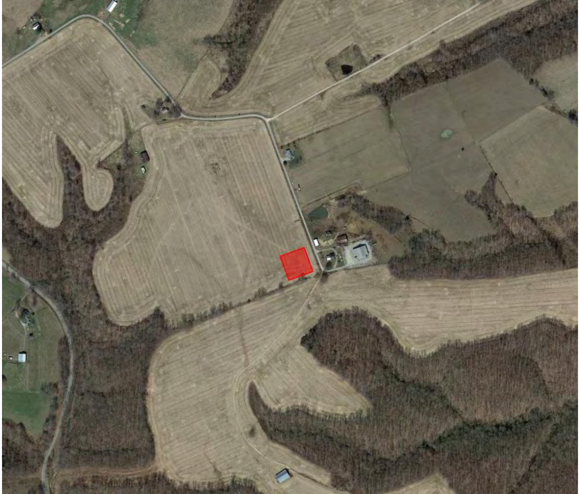
Figure 4: Site of the Proposed EKPC Liberty Power Station with M&R Station Highlighted
