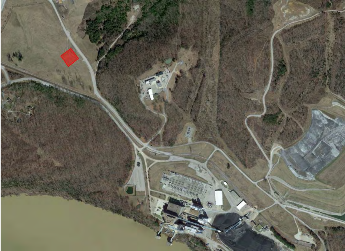
Figure 3: EKPC Cooper Power Station with M&R Station Highlighted
