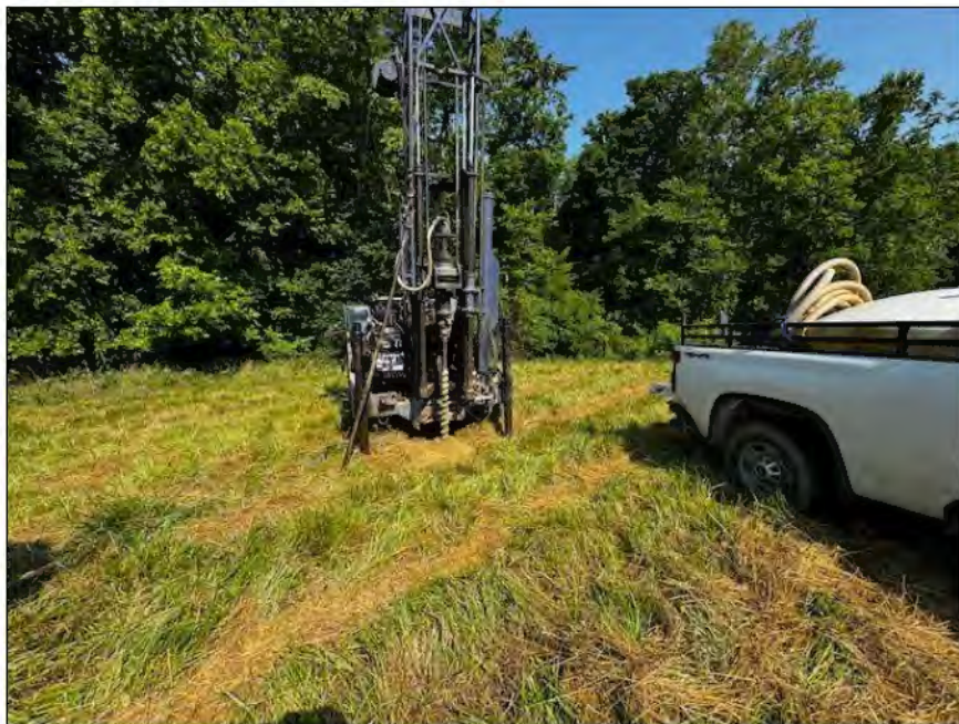
Boring Location at Approximate Tower Center
