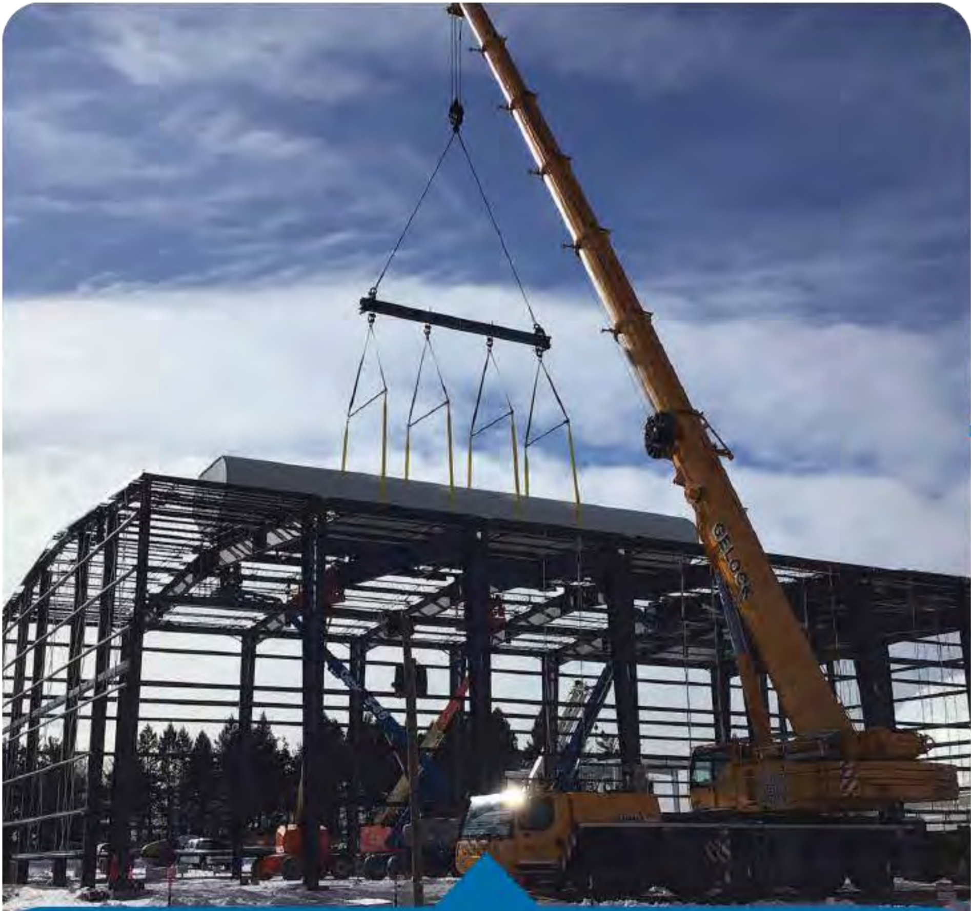
Building Erection 3 months
