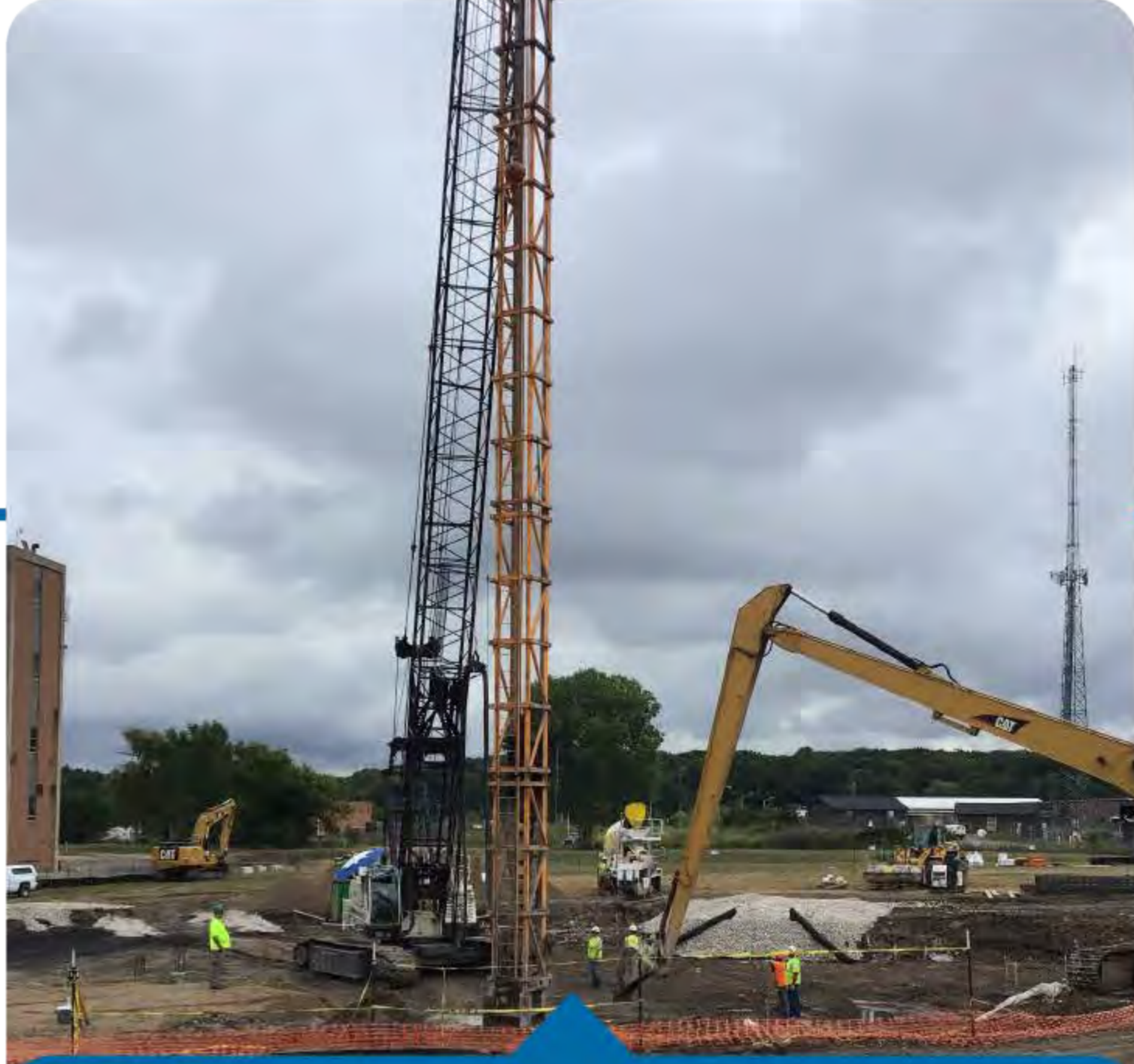
Deep Foundations 2 months
