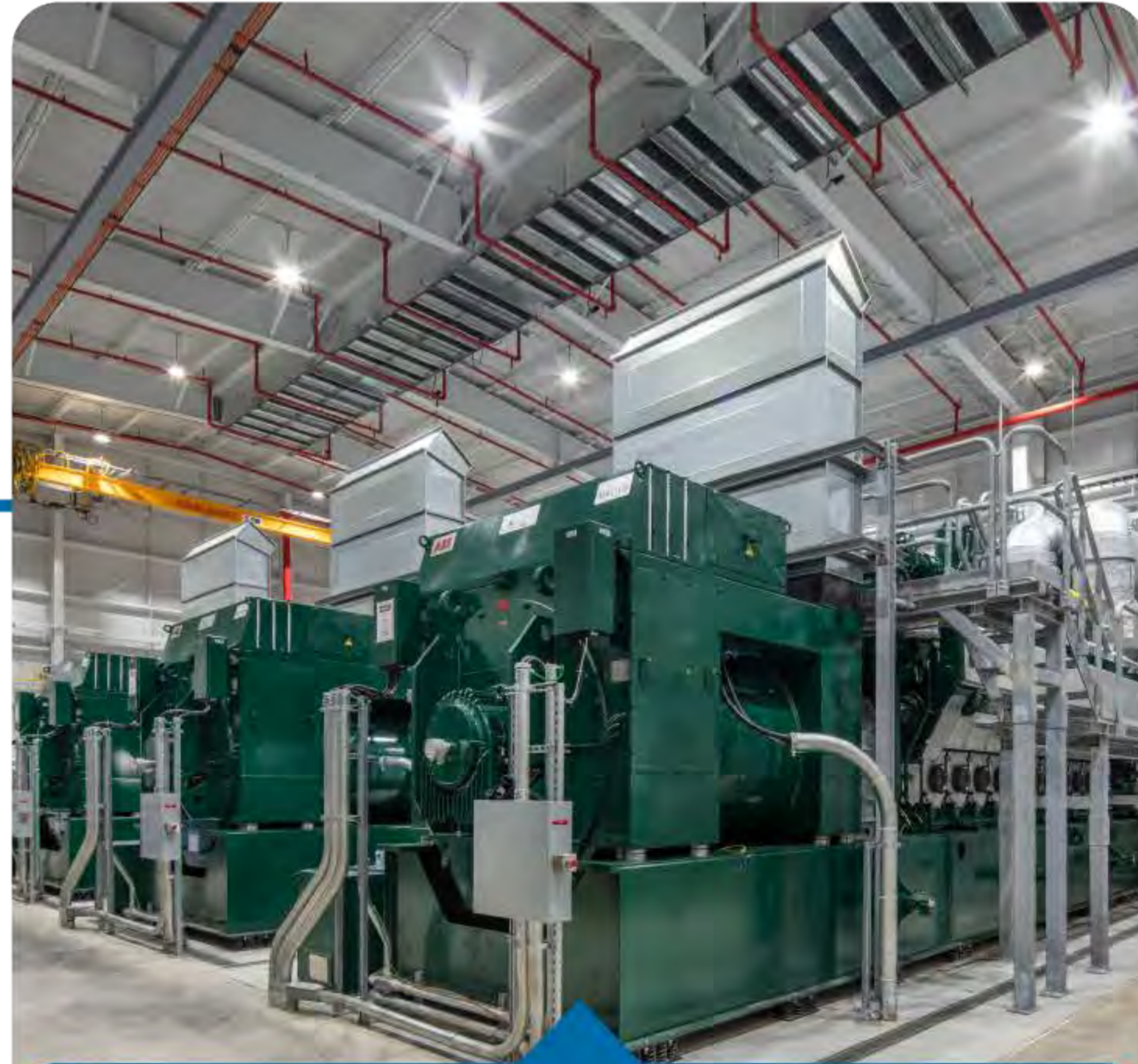
Start-Up + Commissioning 6 months
