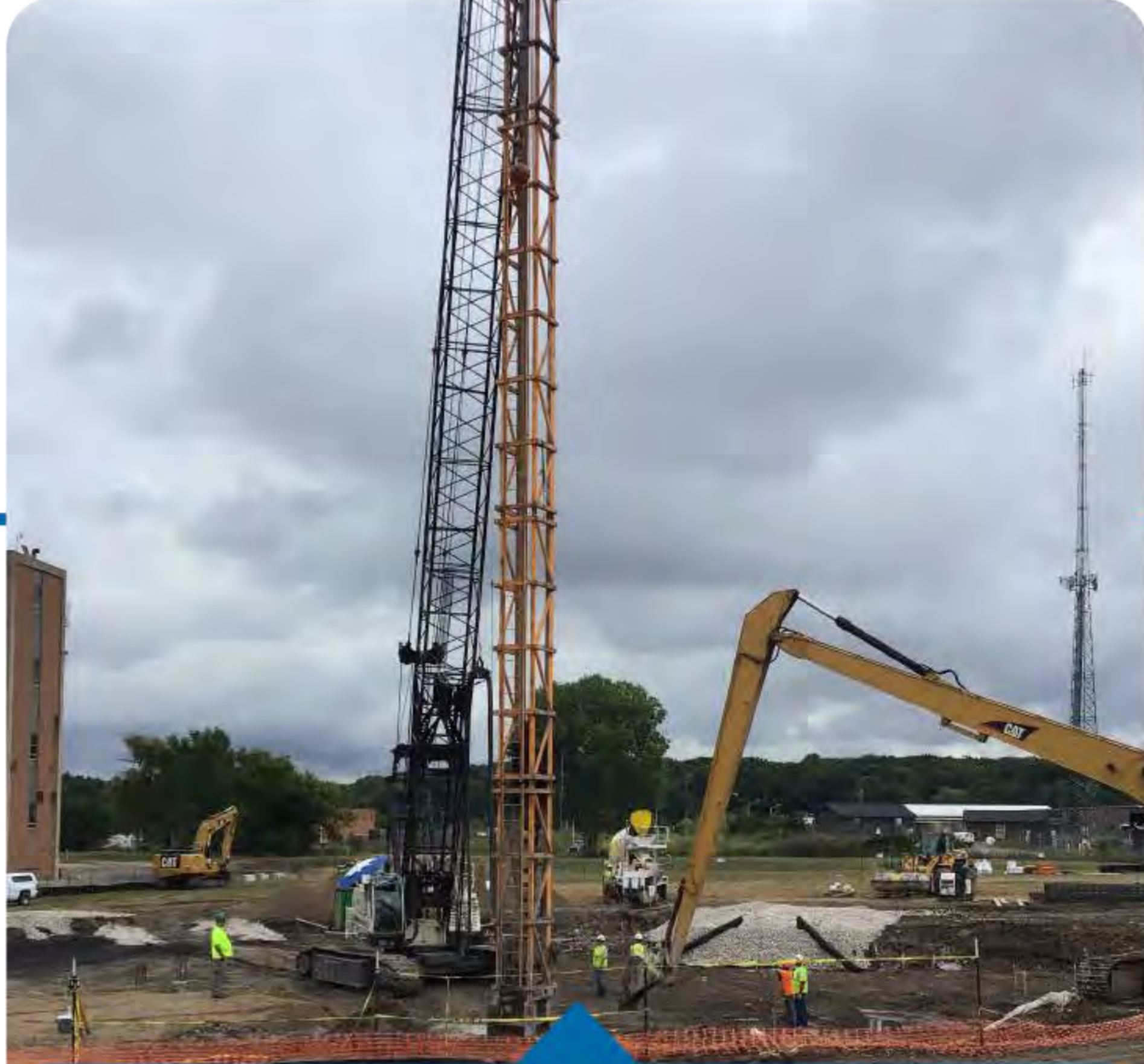
Deep Foundations 2 months
