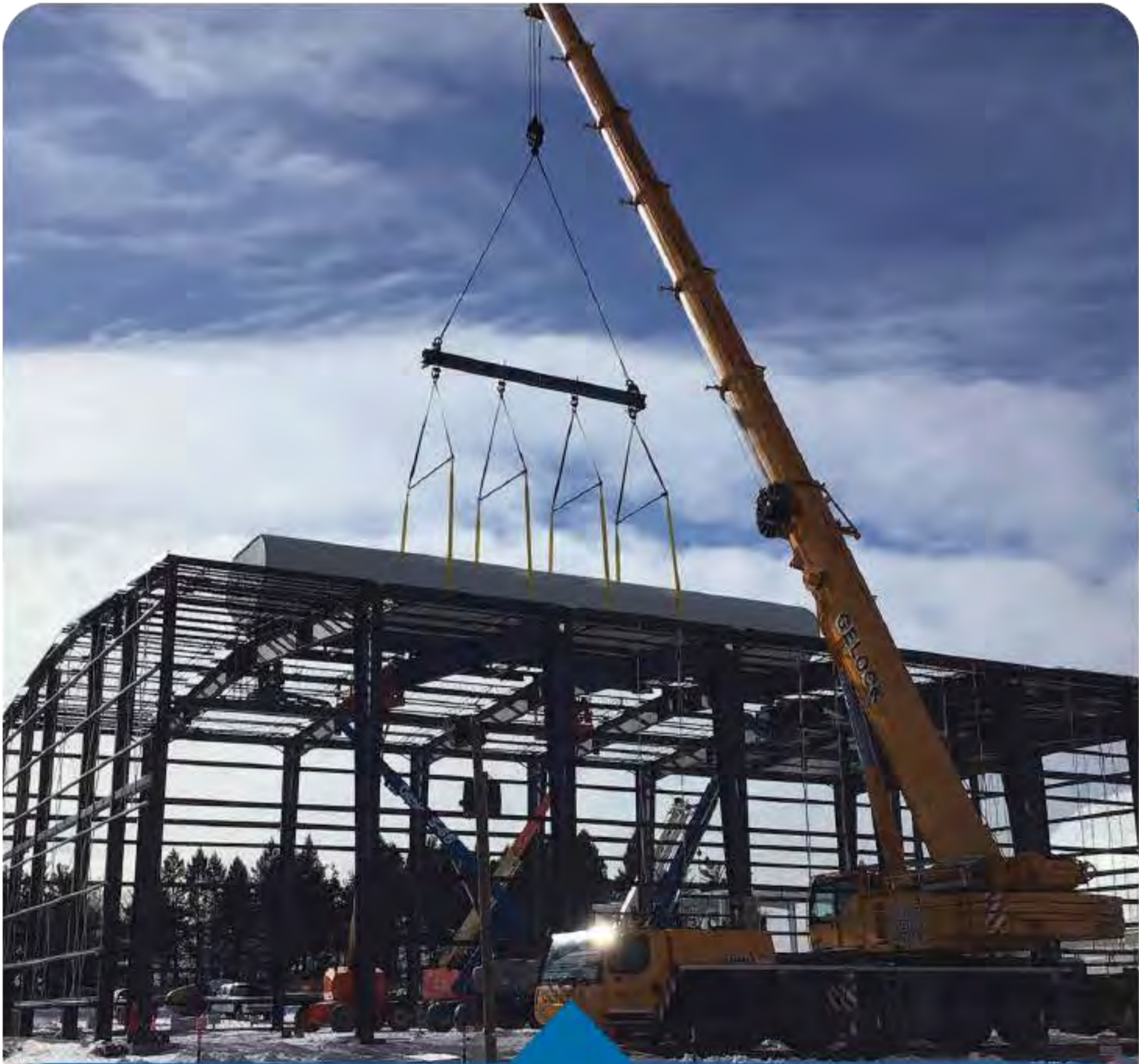
Building Erection 3 months
