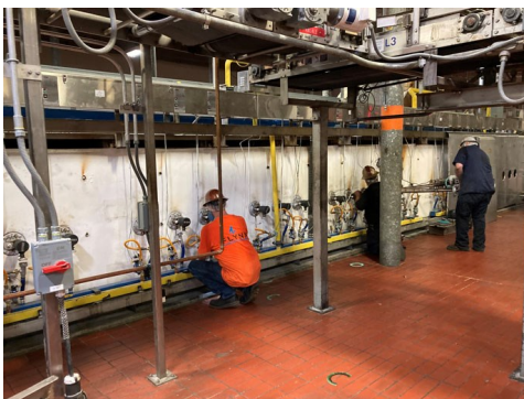
Combi-burners, zone 5 replacement and interior re-firing
