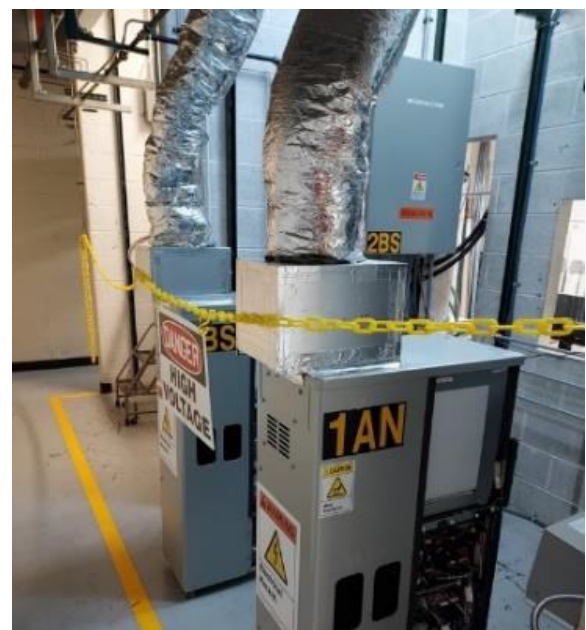
AISIN SOFCs installation at research laboratory
