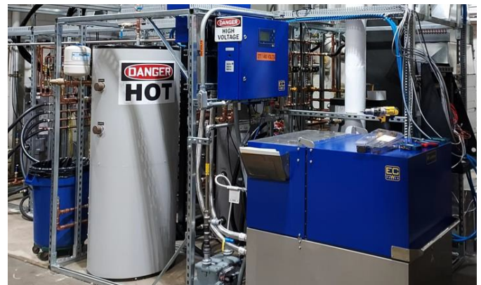
The mCHP integrated system indoor installation.
