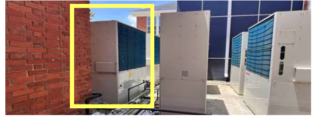
One of seven two-pipe GHPs installed at Pike Road School in Alabama.
