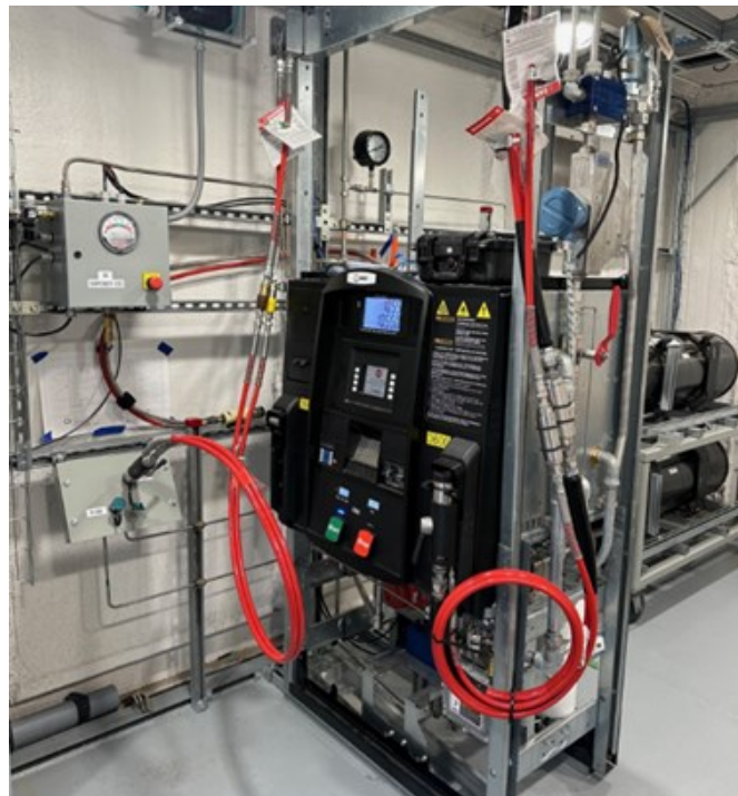
The fully installed ANG1 dispenser
