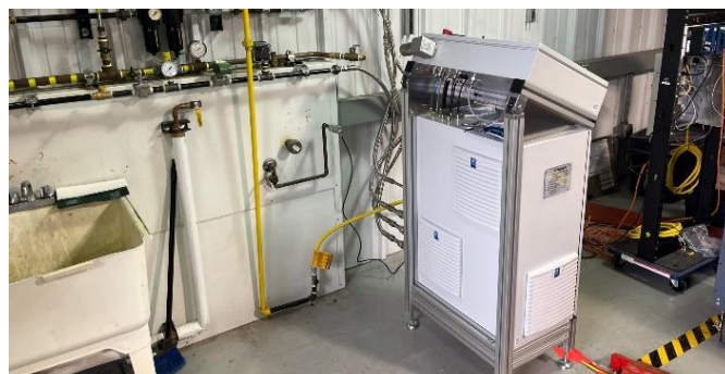
H2 Source and Mixer Undergoing Installation
