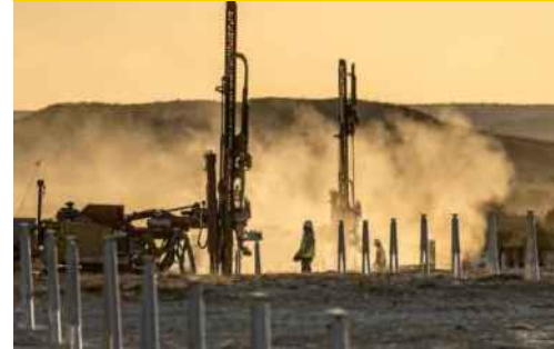
Foundation & Racking Installation
