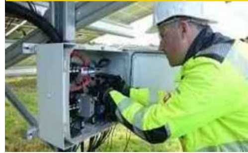
Final Testing & Landscaping
