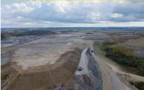
Grading & Site Prep
