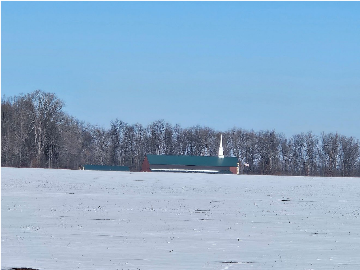
Figure C-14. New Hardinsburg Baptist Church Behind Future Array Area
