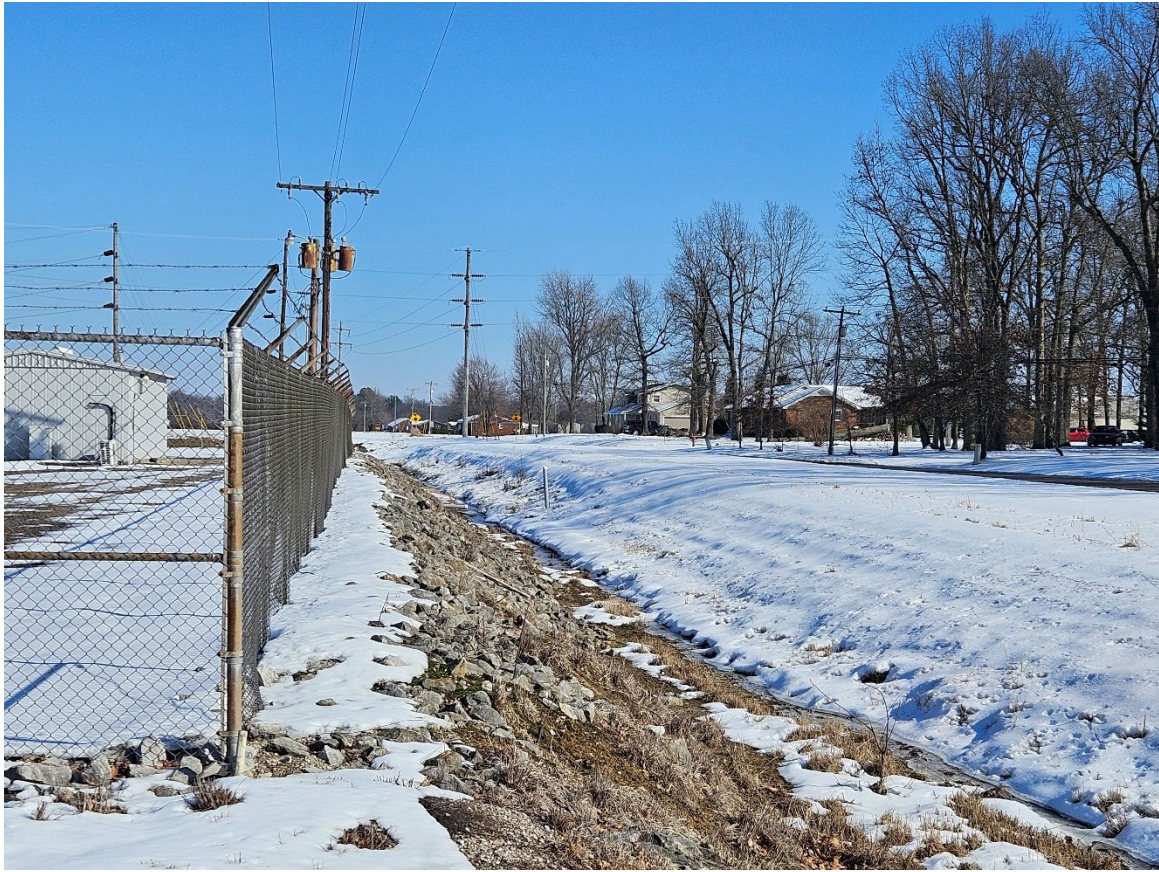
Figure C-18. Quail Run Neighborhood Near Substation
