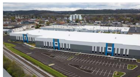
The new 146,000 square foot industrial building that Thermo Fisher Scientific will call home. Photo provided | BE NKY Growth Partnership
