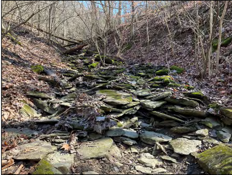
Photograph 23: View of intermittent S-17, facing east.
