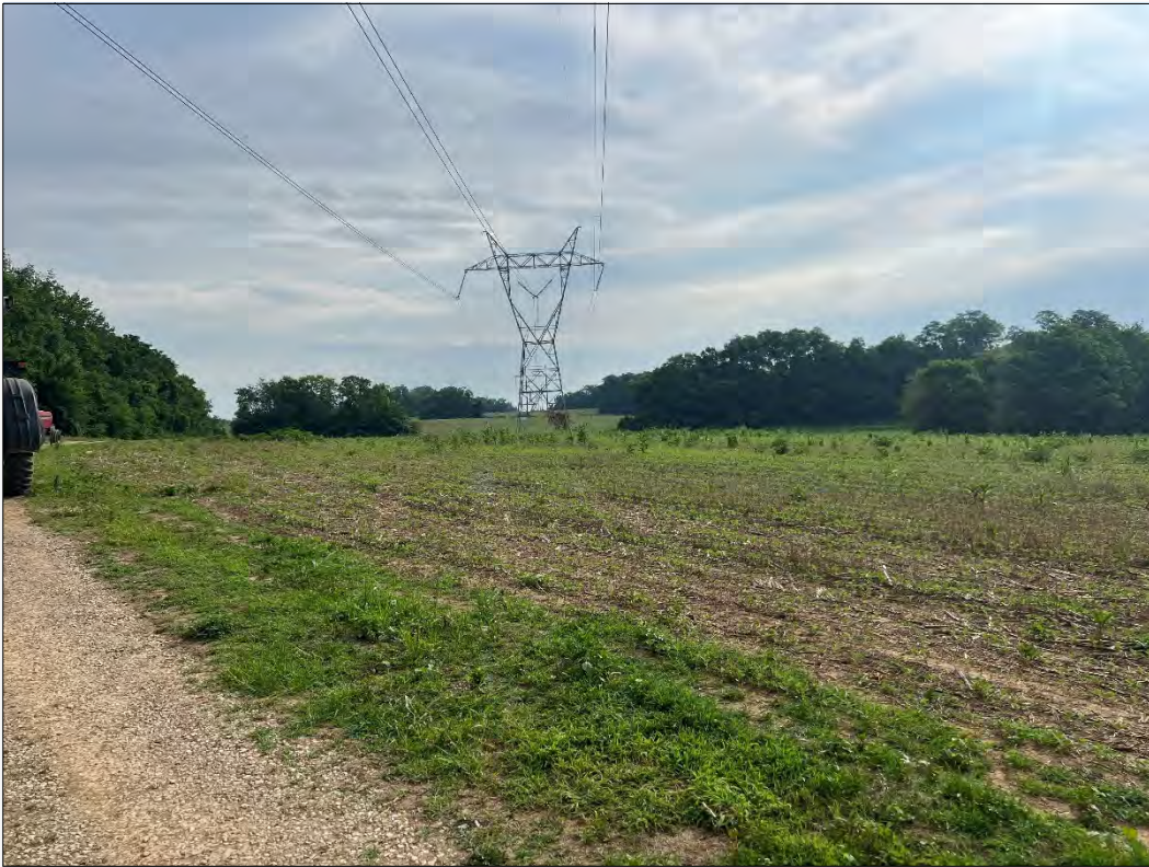
Photograph 10. View of EKPC's Spurlock – Avon 345 kV transmission line
