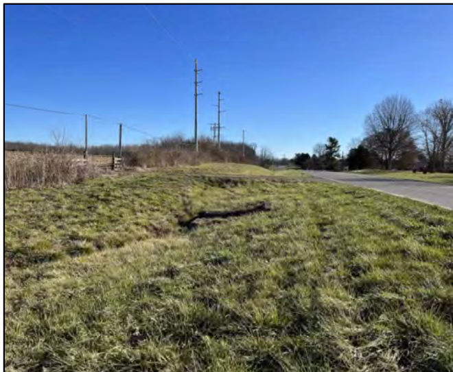
Figure 1. Near Access Point #1 Looking East at US 60
