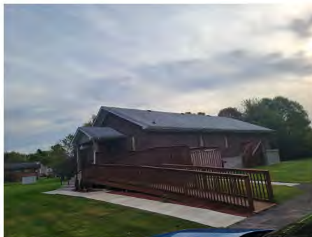
Figure 24: Built Avoidances within the Project AOI (NV5 Field Survey)
