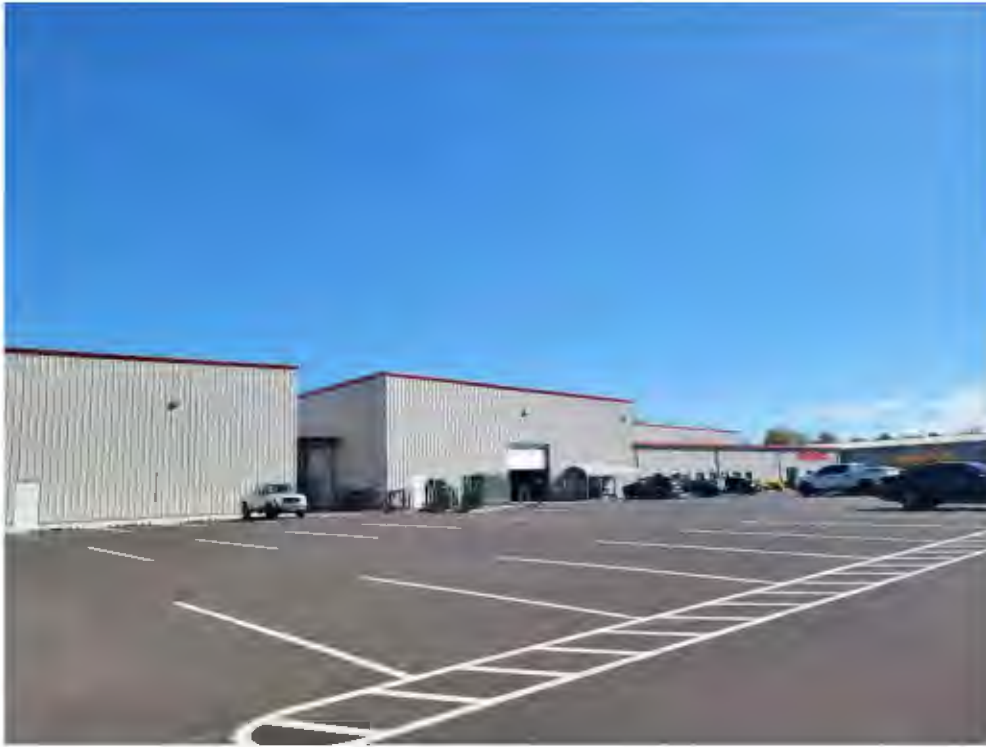
Figure 18: Building within the AOI (NV5 Field Photo)
