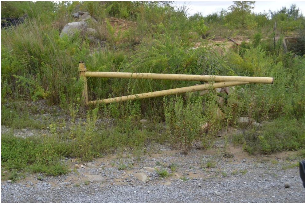
Site Entrance Gate Location, Top of Access Road from Brushy Road
