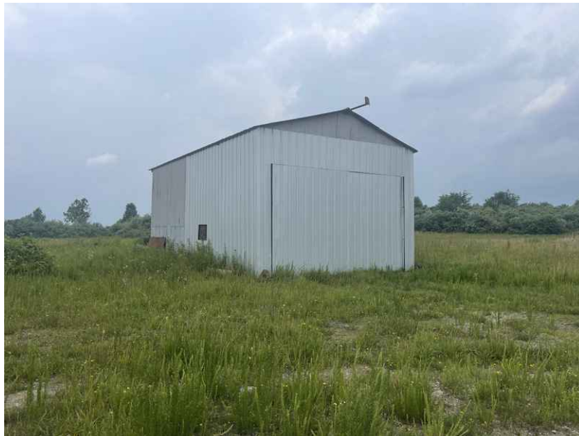
View of the steel structure on the eastern portion of the Subject Property
