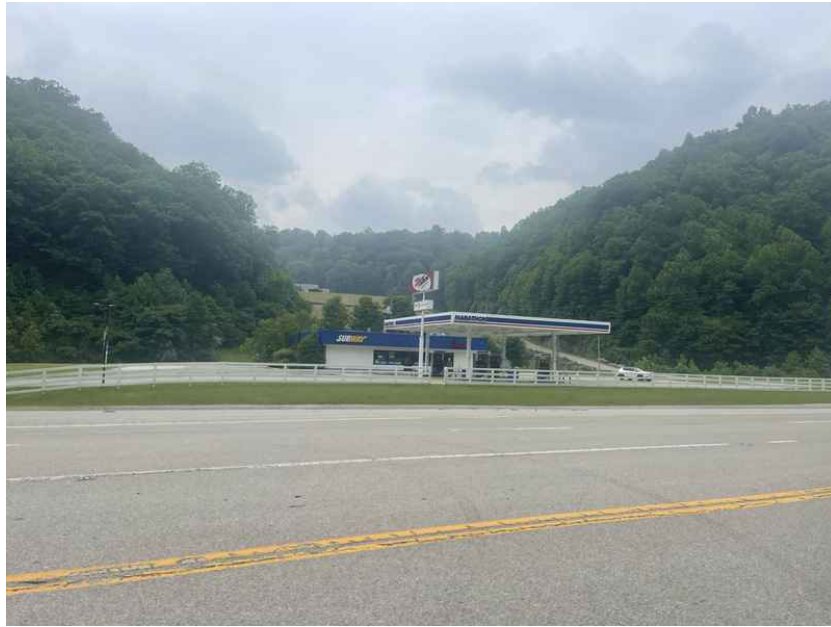
View of the Exon Mobil gas station, situated west of the Subject Property
