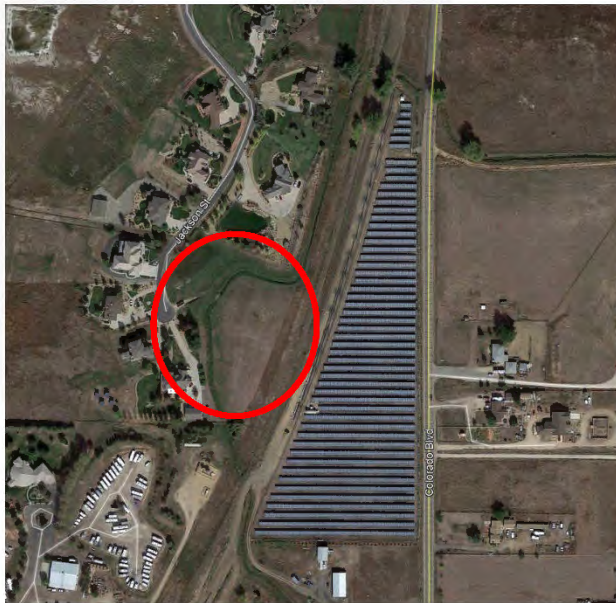
Brighton PV Solar, Adams County, CO June 2016
