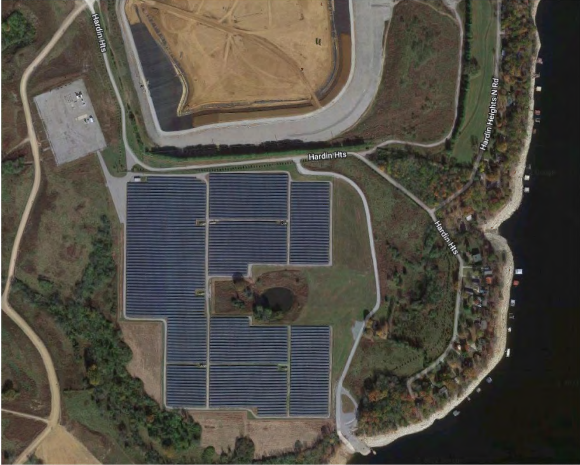
E.W. Brown Generating Station Solar Field
