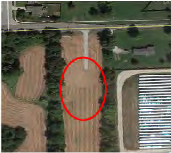
Dominion Indy III Solar Farm September 2014
