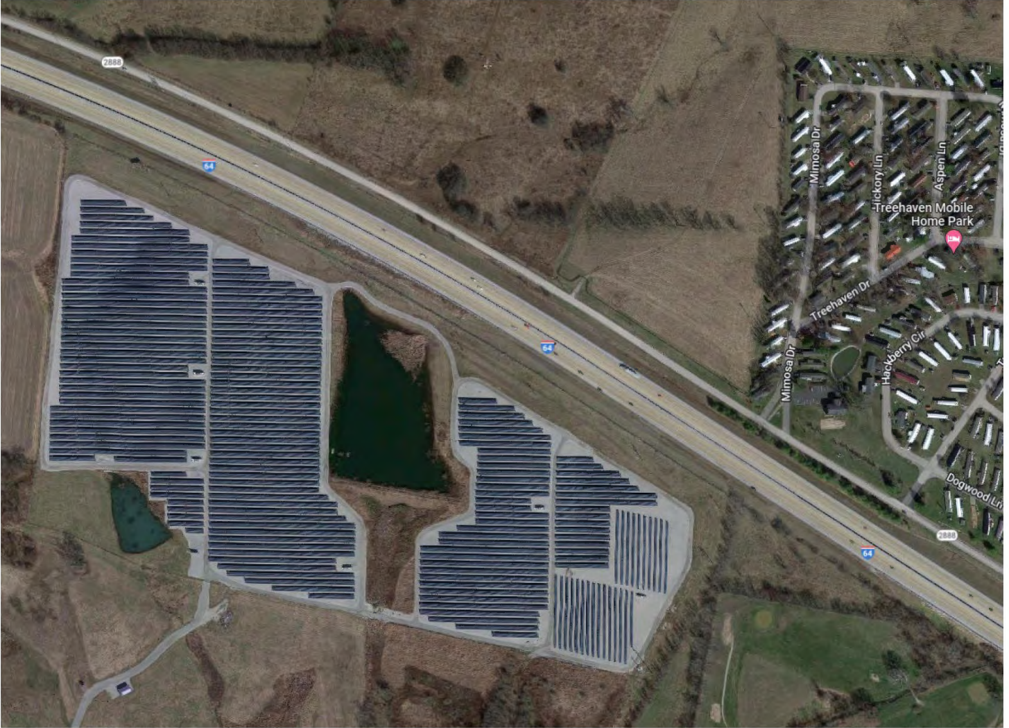
East KY Power Coop Solar Field
