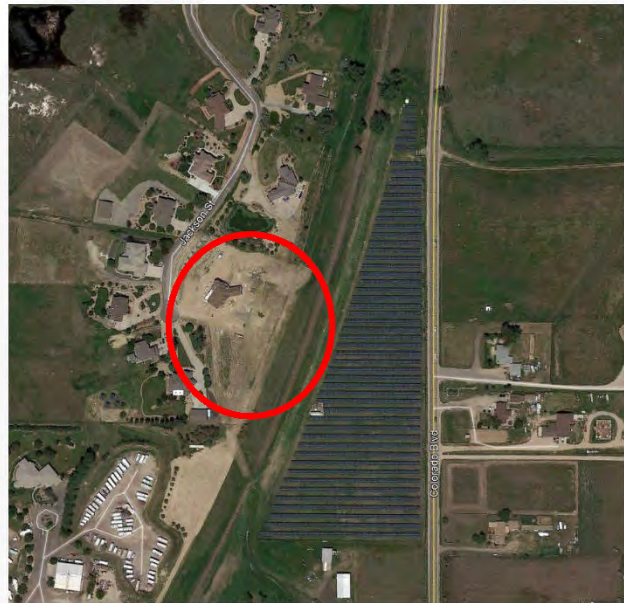
Brighton PV Solar, Adams County, CO June 2017
