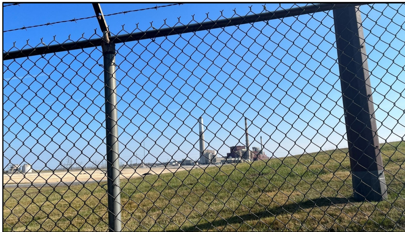
Proposed Project/BESS Facility View from Dix Dam Road/Hardin Heights Road
