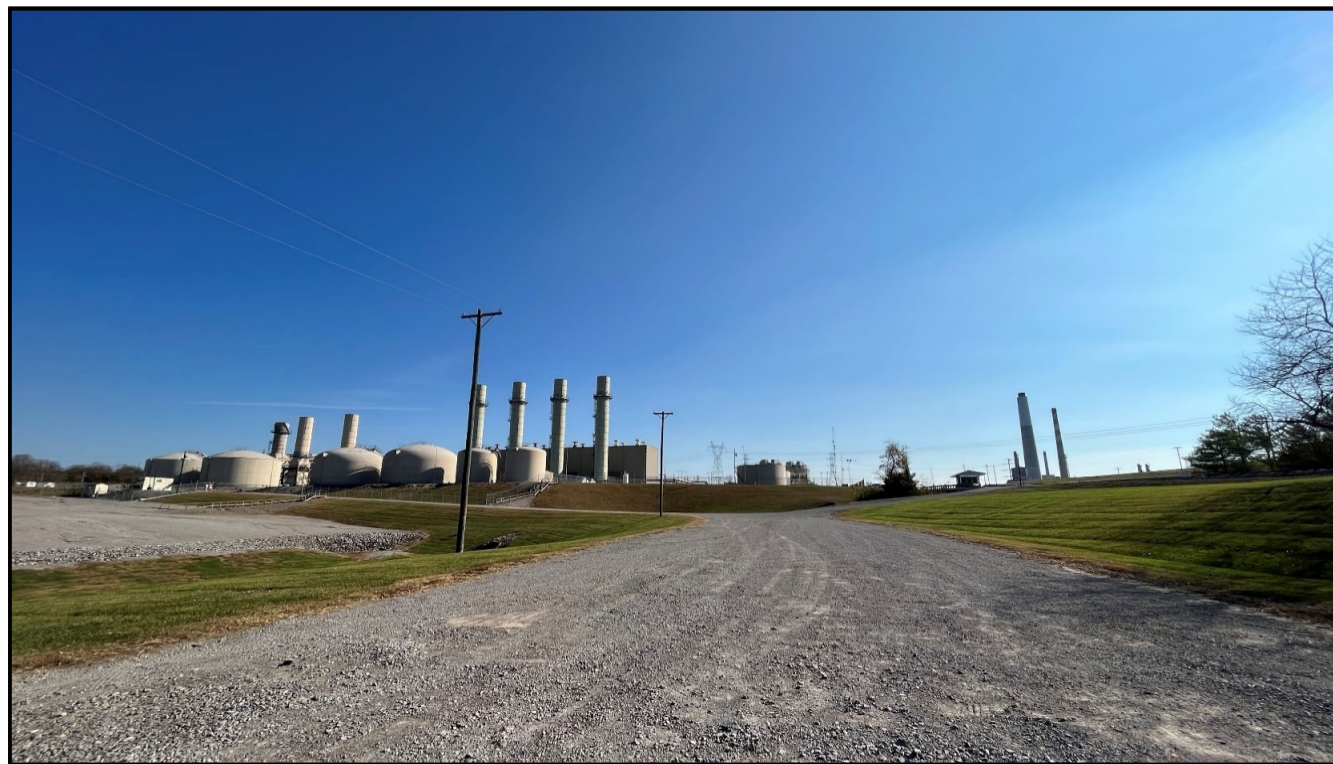
Proposed Project/BESS Facility View from E.W. Brown Station Main Entrance
