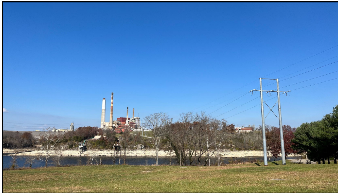
Proposed Project/BESS Facility View from Hunter Drive/Domar Drive
