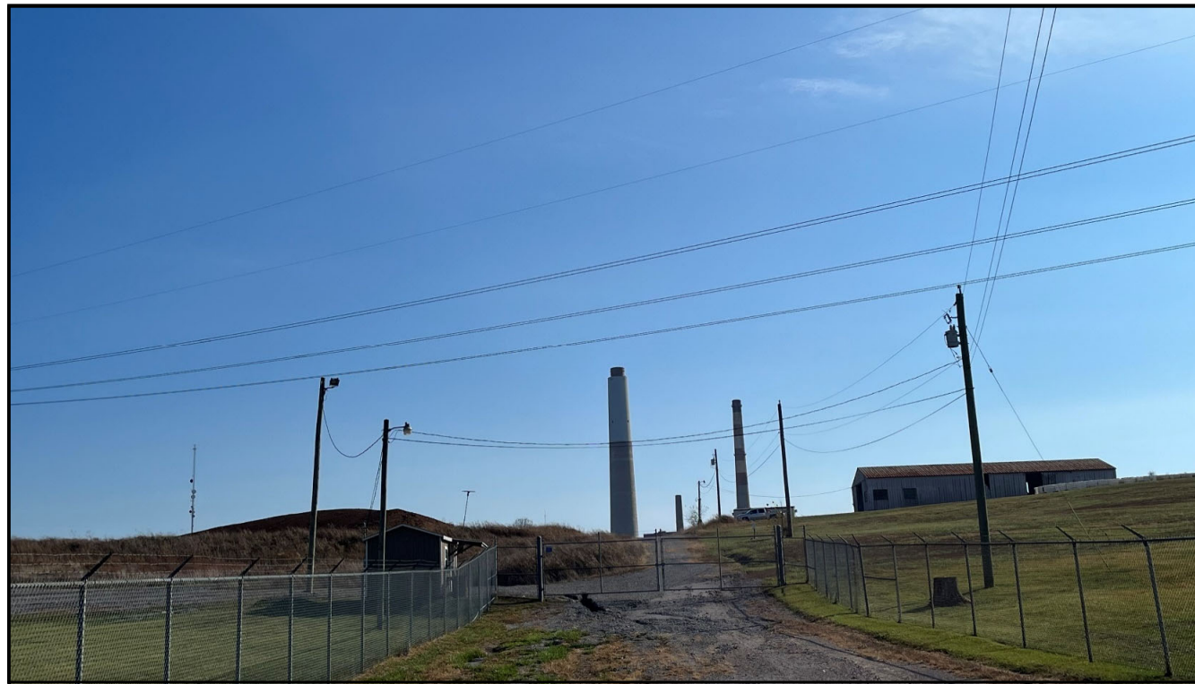
Proposed Project/BESS Facility View from Brown Station Secondary Entrance (Gate 5)
