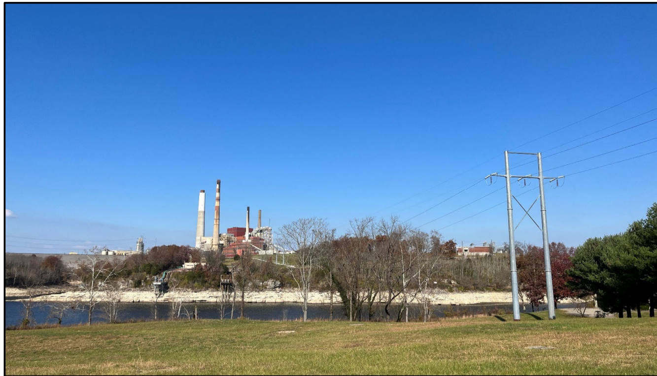
Existing/Baseline View from Hunter Drive/Domar Drive
