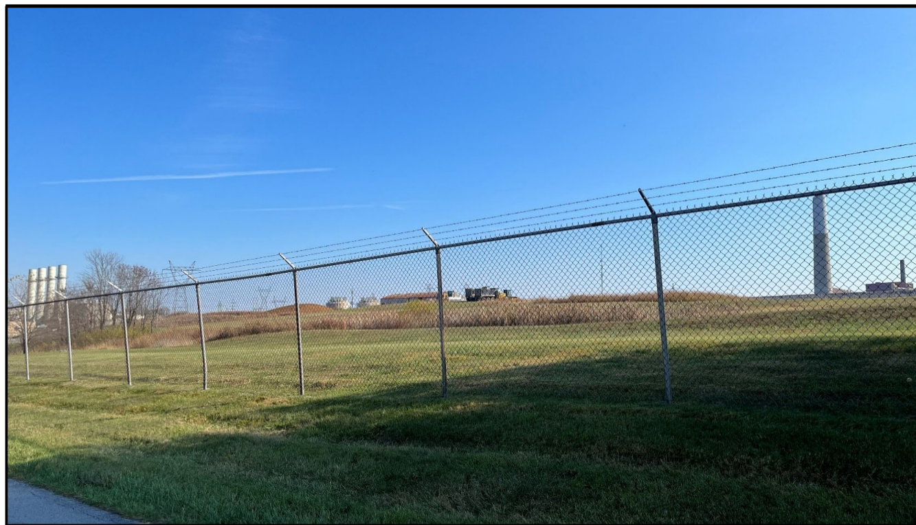
Proposed Project/BESS Facility View from Dix Dam Road
