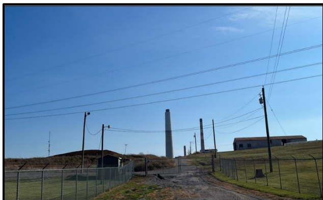
Photo Location #3: Looking east from Brown Station's secondary (Gate 5) facility entrance along Dix Dam Road.
