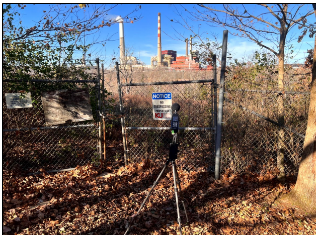
Photo Location #3: Brown Station southern existing property boundary – Hardin Heights North Road.
