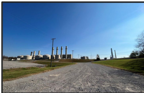
Photo Location #4: Looking southeast from the Brown Station main entrance along Dix Dam Road.
