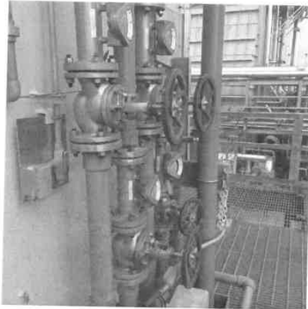
Evaporative Cooler Tuning Valves (x4)
