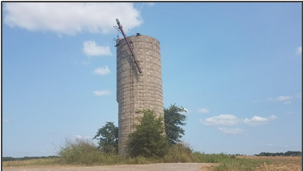
Figure 15. Silo in the location of MS 25, facing northeast.
