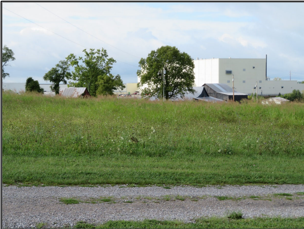
Figure 14. ME 504: Barns and outbuildings, looking south-southwest.
