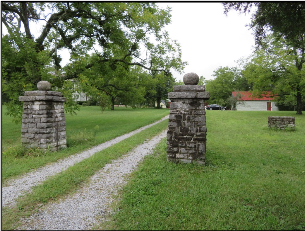
Figure 8. ME 170: Contributing outbuildings associated with ME 170, looking north.
