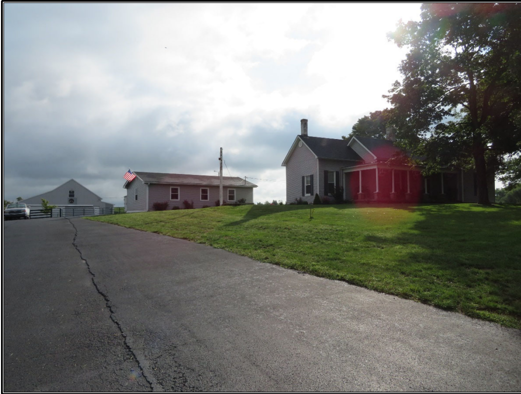
Figure 17. ME 507: House and outbuildings, looking northeast.
