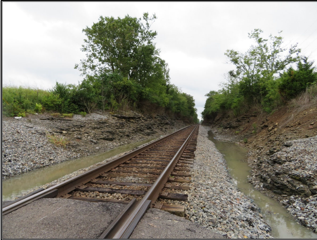
Figure 21. ME 510: Railroad leading to culvert, looking south.
