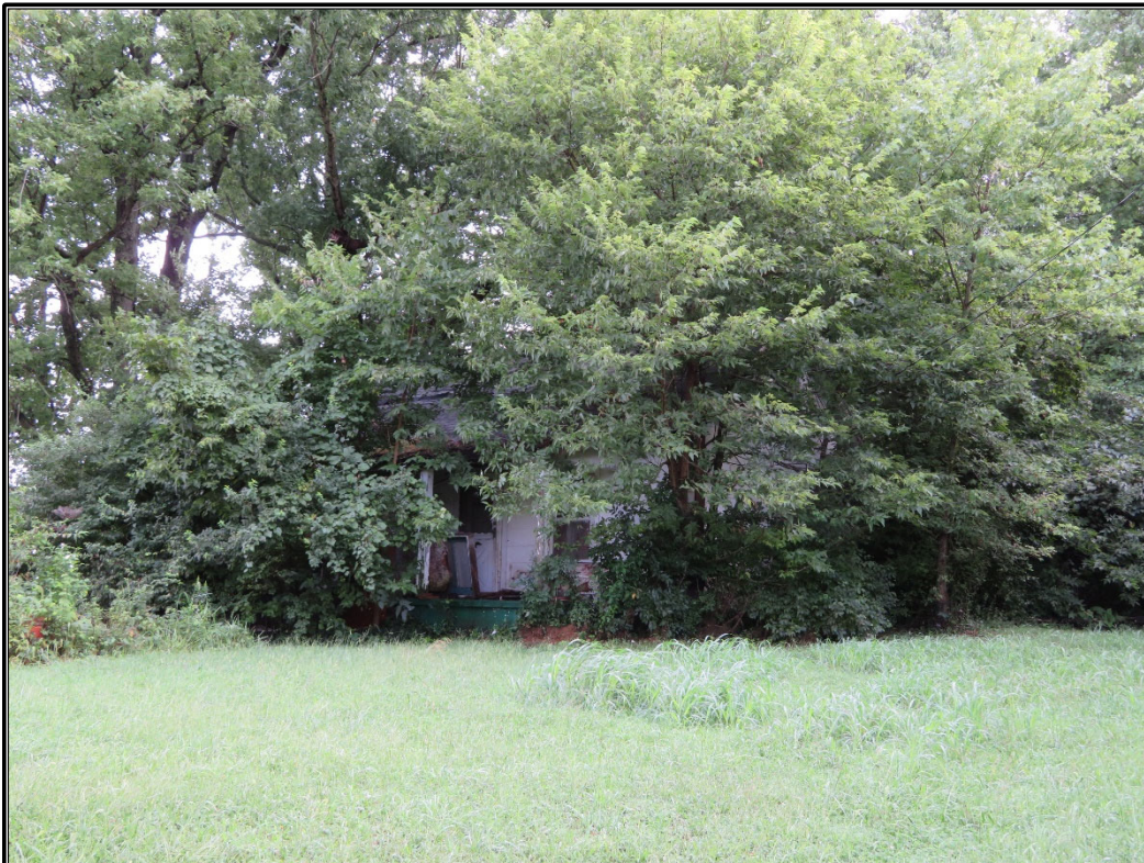
Figure 16. ME 506: Vacant house, looking north-northeast.
