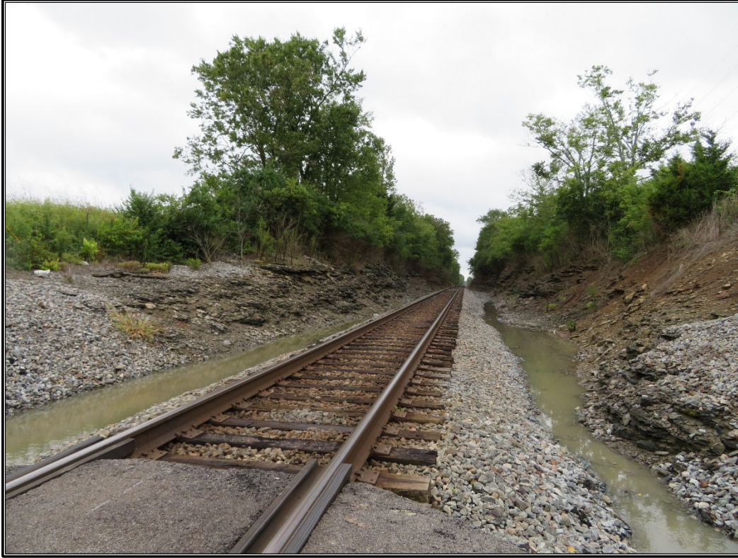
Figure 37. ME 539: View towards trestle, looking south.
