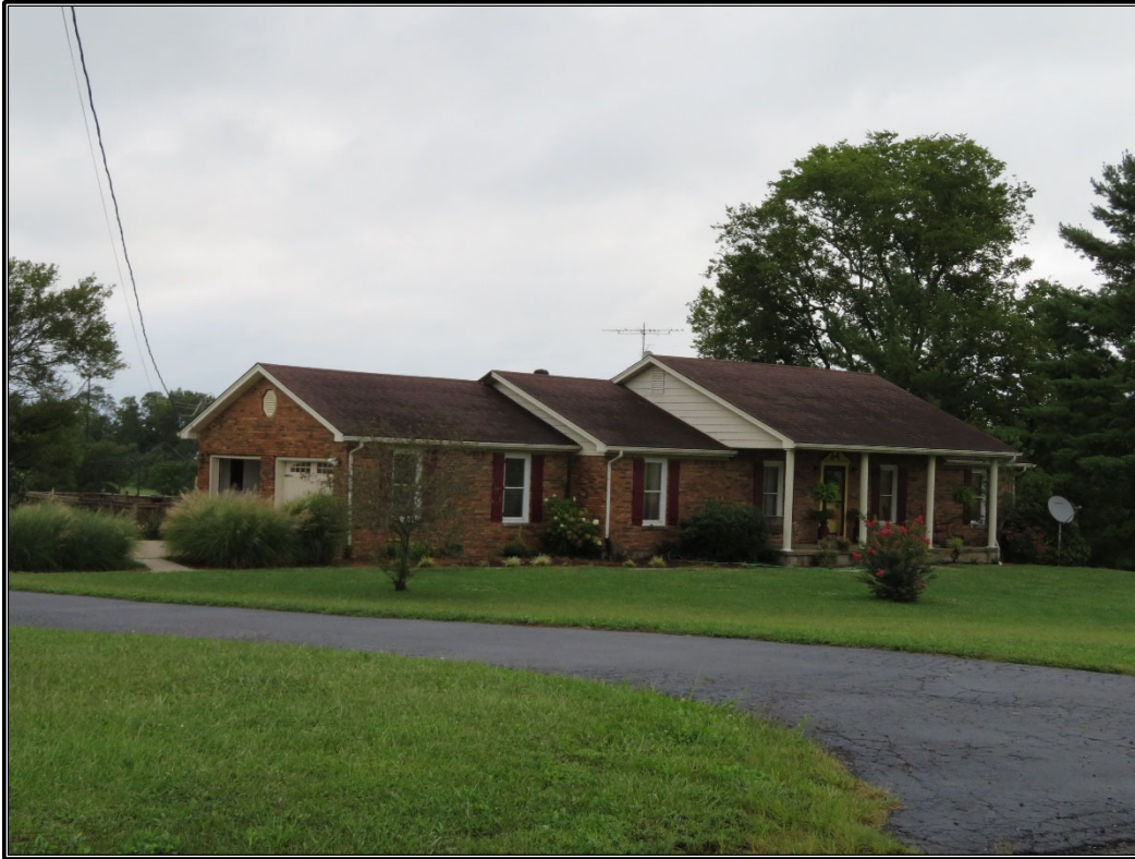
Figure 33. ME 513: Non-historic house, looking northeast.
