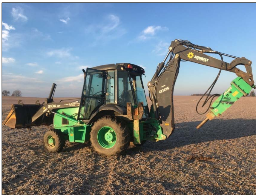
Excavator and Vibratory Hammer Used for Post Installation
