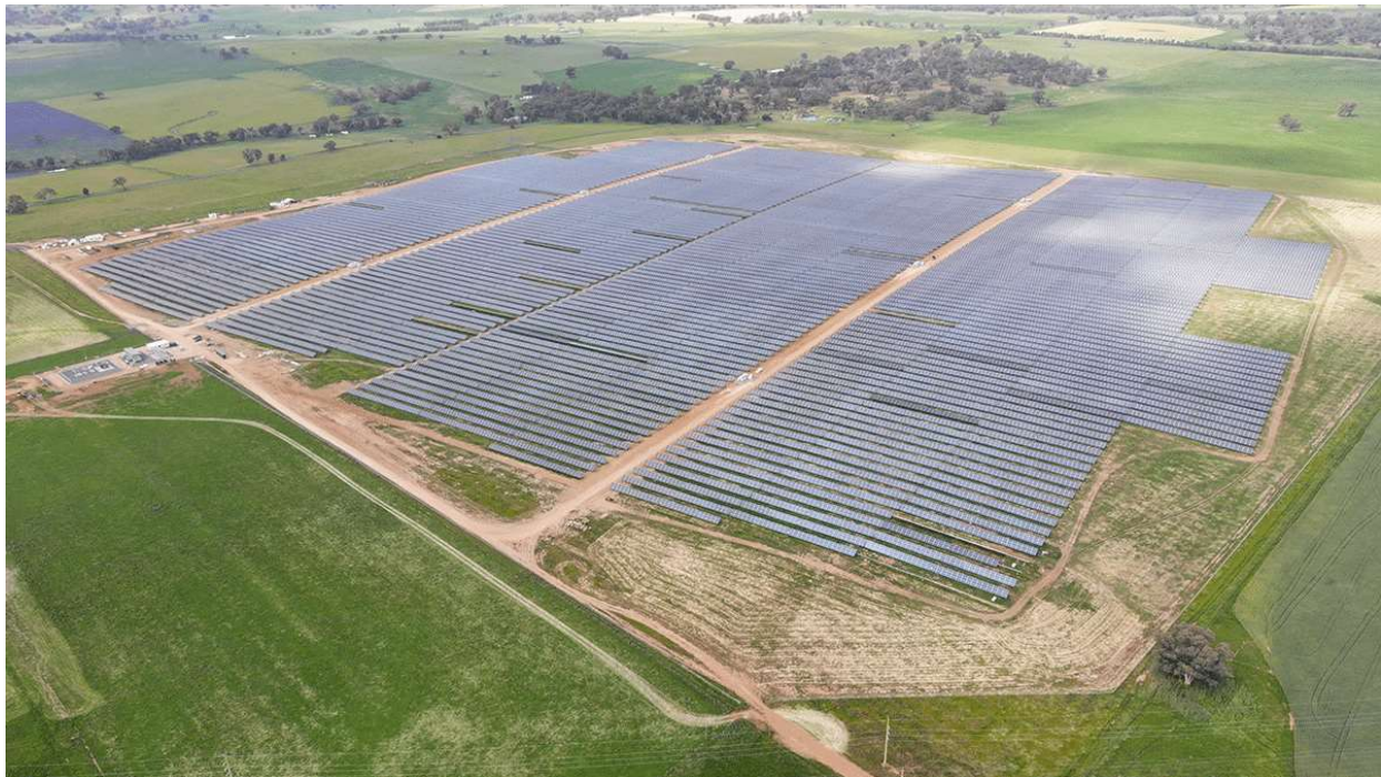
Picture (3) Solar Modules Installed on Farmland 3
