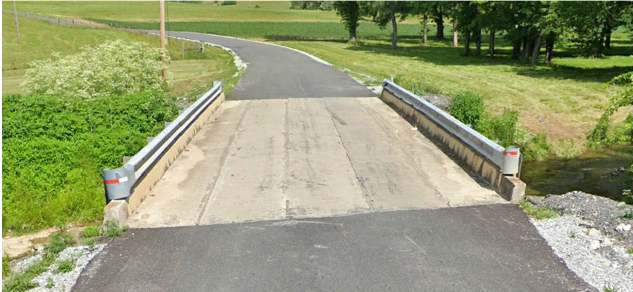
Picture (50) Bridge along Booker Road (NBI: 115C00047N)
