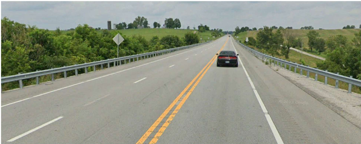
Picture (48) Bridge along Springfield Highway (KY-55) (NBI: 115B00048N)
