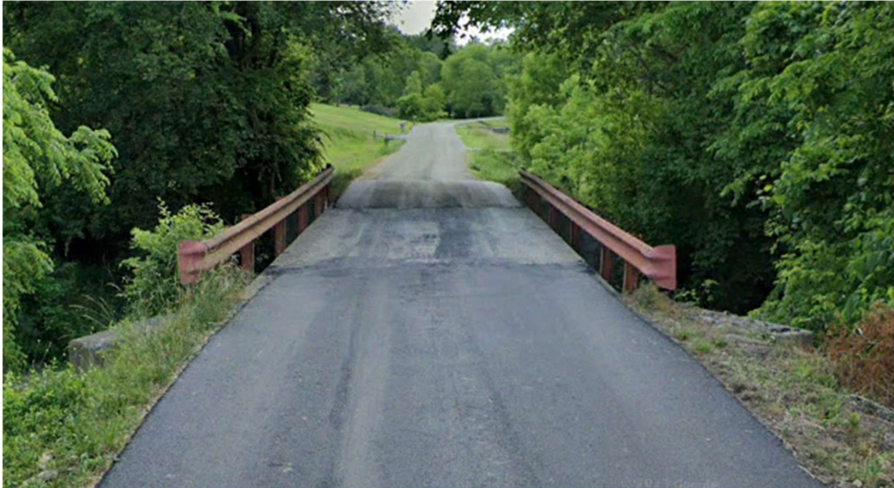
Picture (44) Bridge Radio Station Road (NBI: 078C00126N)
