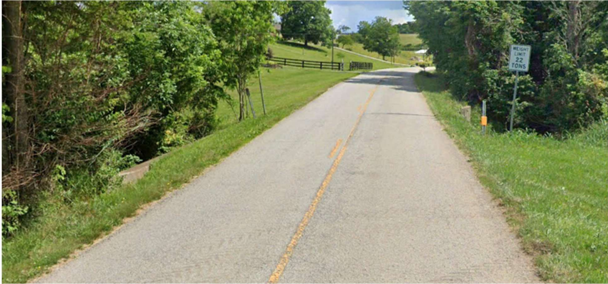
Picture (47) Bridge along St. Rose Road (NBI: 115B00018N)
