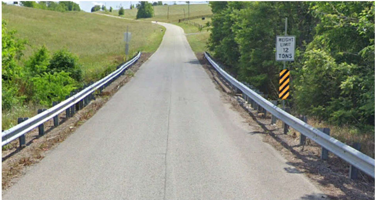
Picture (46) Bridge along Old Lebanon Road (NBI: 115B00017N)
