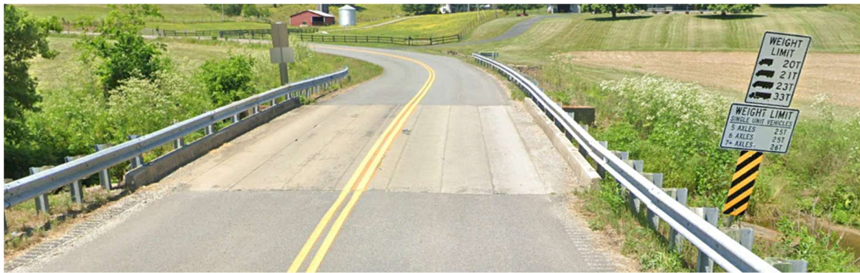
Picture (41) Bridge along St. Rose Road (NBI: 078B00062N)
