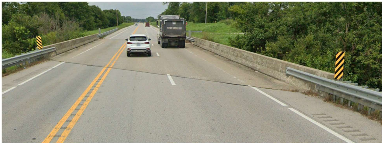
Picture (42) Bridge along Springfield Highway (KY-55) (NBI: 078B00069N)
