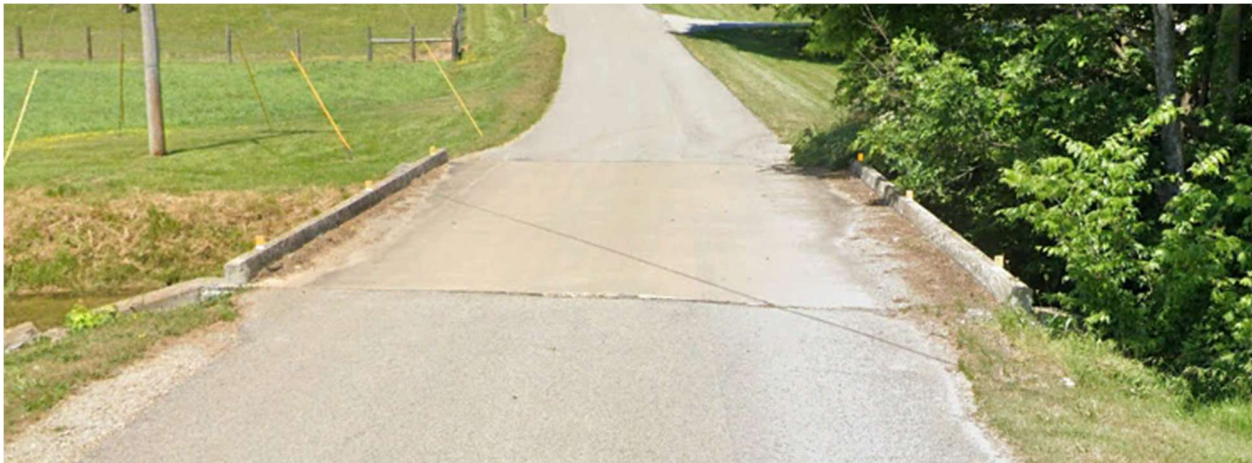
Picture (51) Bridge along Smith Lane (NBI: 115C00061N)
