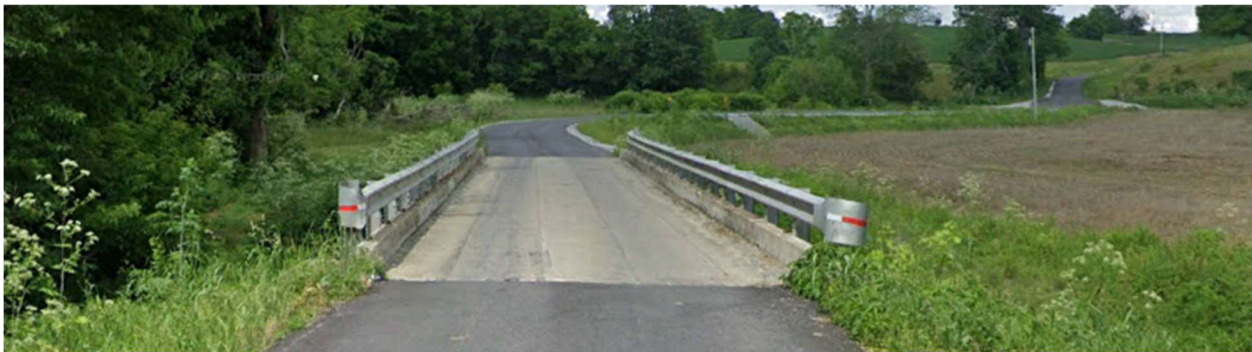
Picture (49) Bridge along Booker Road (NBI: 115C00041N)
