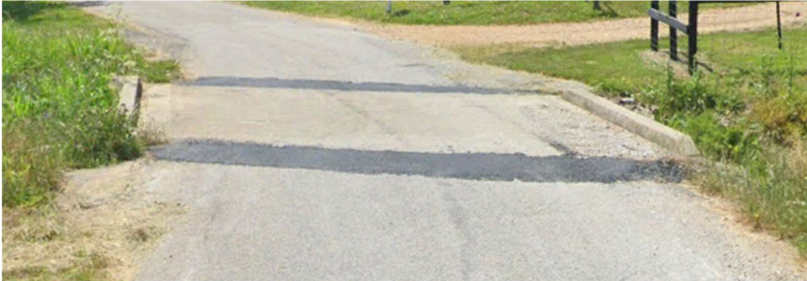
Picture (43) Bridge along Horan Lane (NBI: 078C00102N)
