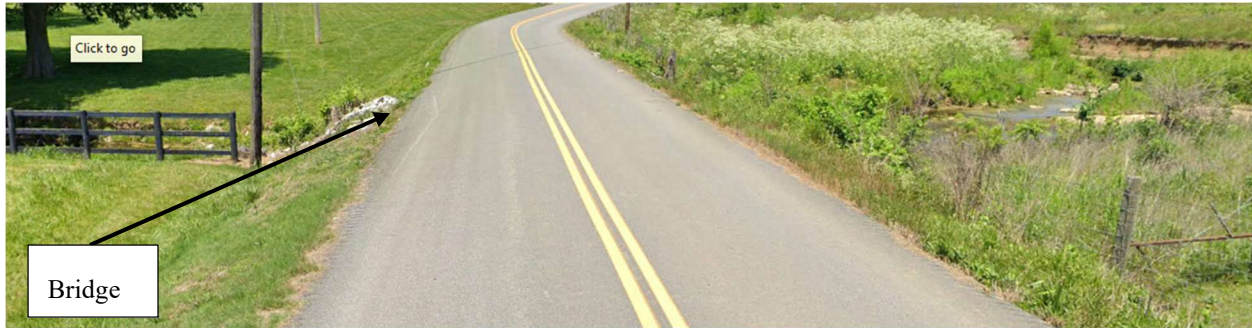
Picture (40) Bridge along St. Rose Road (NBI: 078B00050N)
