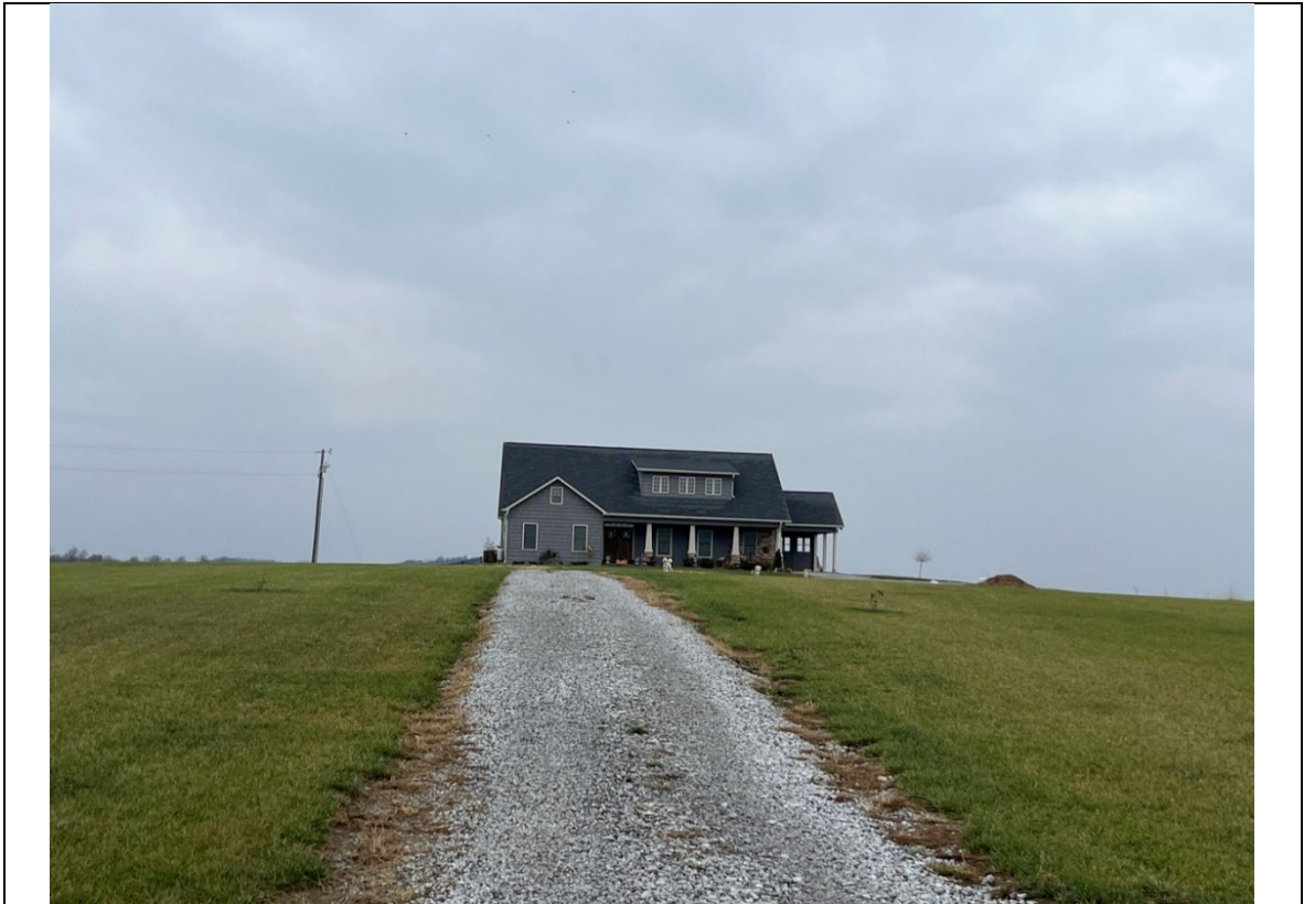
Photograph: 18 | View of the easternmost residence and a pole-mounted transformer.
