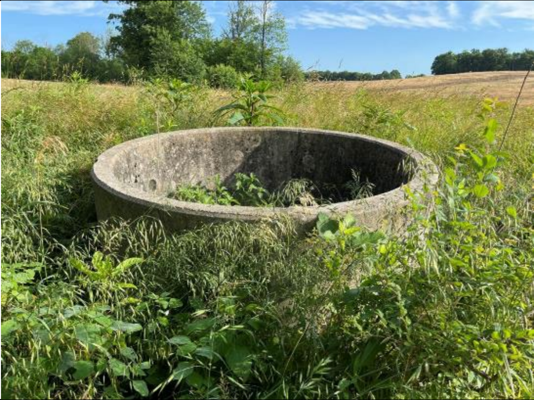
Photograph: 7 | View of a concrete cattle watering hole.
