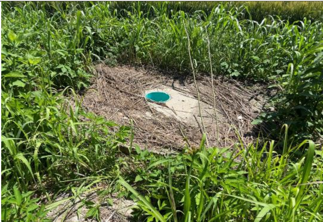
Photograph: 4 | View of groundwater well.
