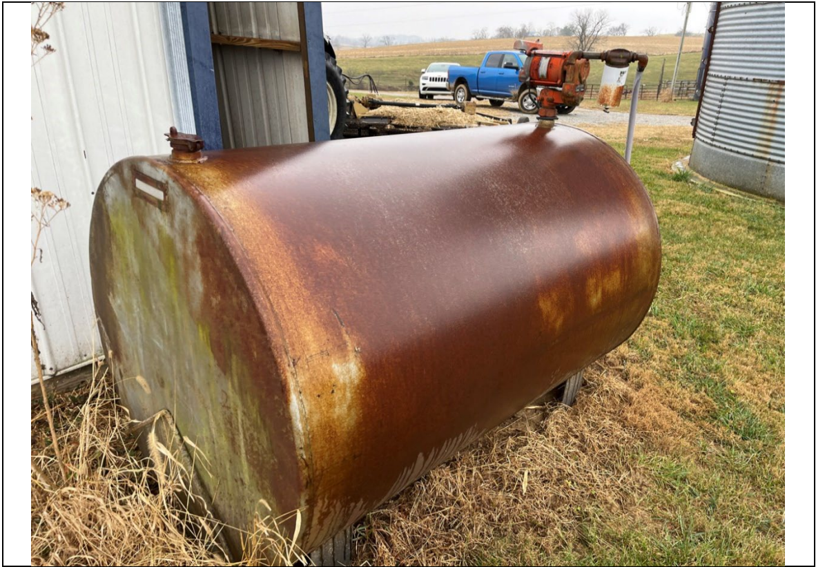
Photograph: 9 | View of an AST located within the northern portion of the Site.
