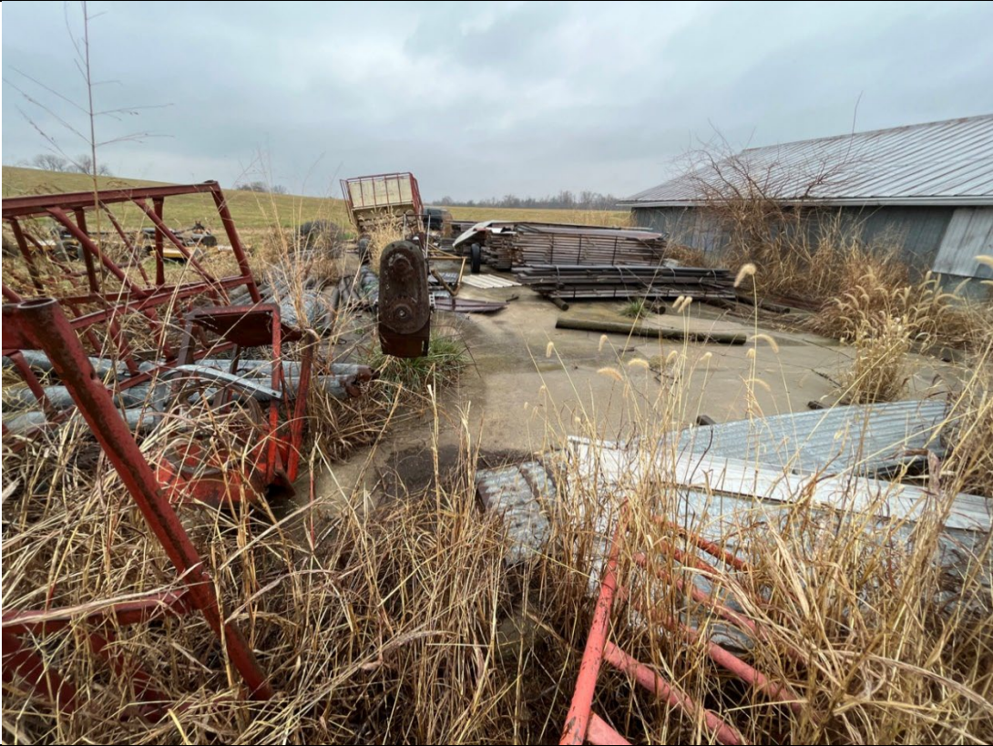
Photograph: 21 | View of a concrete foundation with equipment and building materials.
