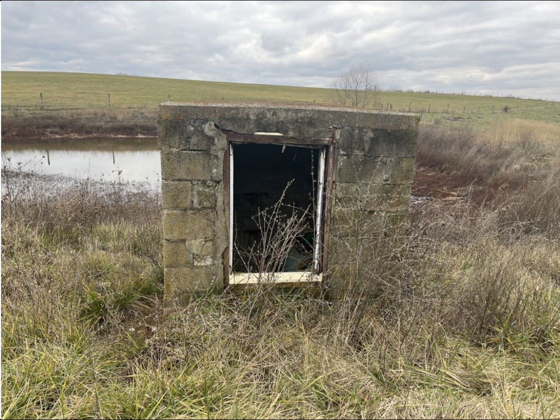
Photograph: 29 | View of well house.
