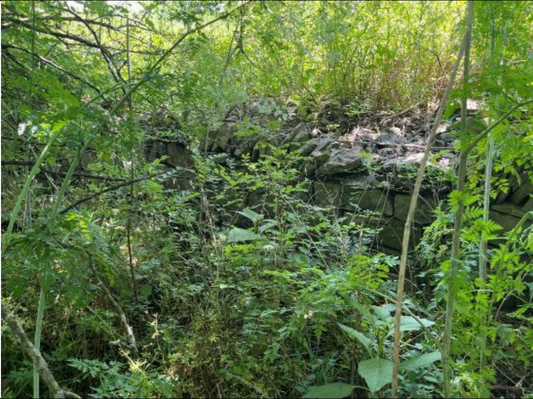
Photograph: 11 | View of the former building foundation.
