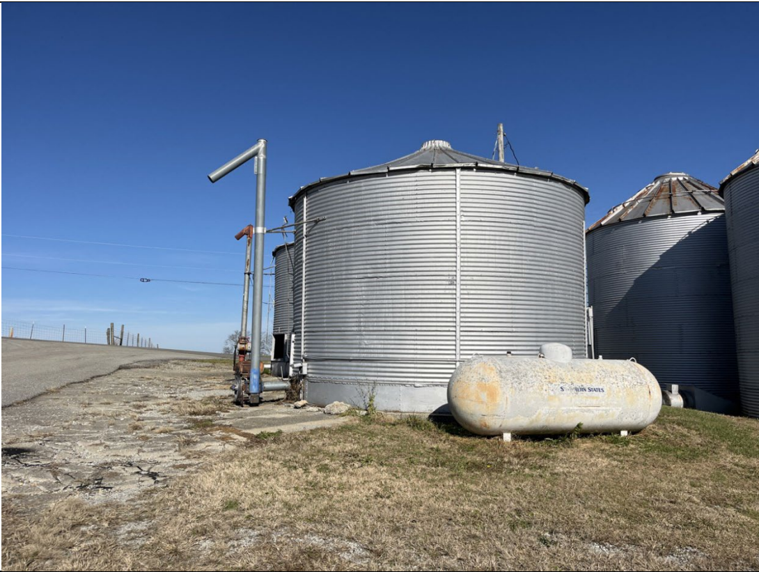
Photograph: 27 | View of silos with AST along McLain Rd.
