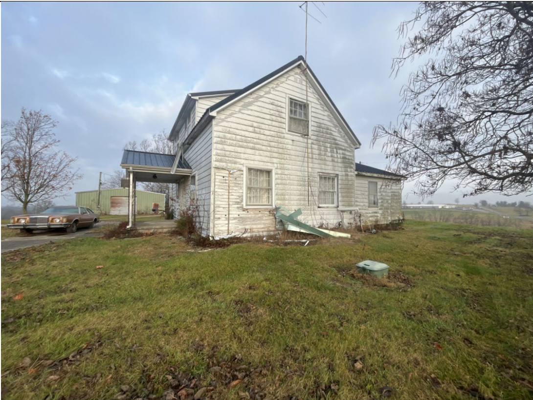
Photograph: 37 | View of residence and barn with underground utilities, Lebanon Rd.
