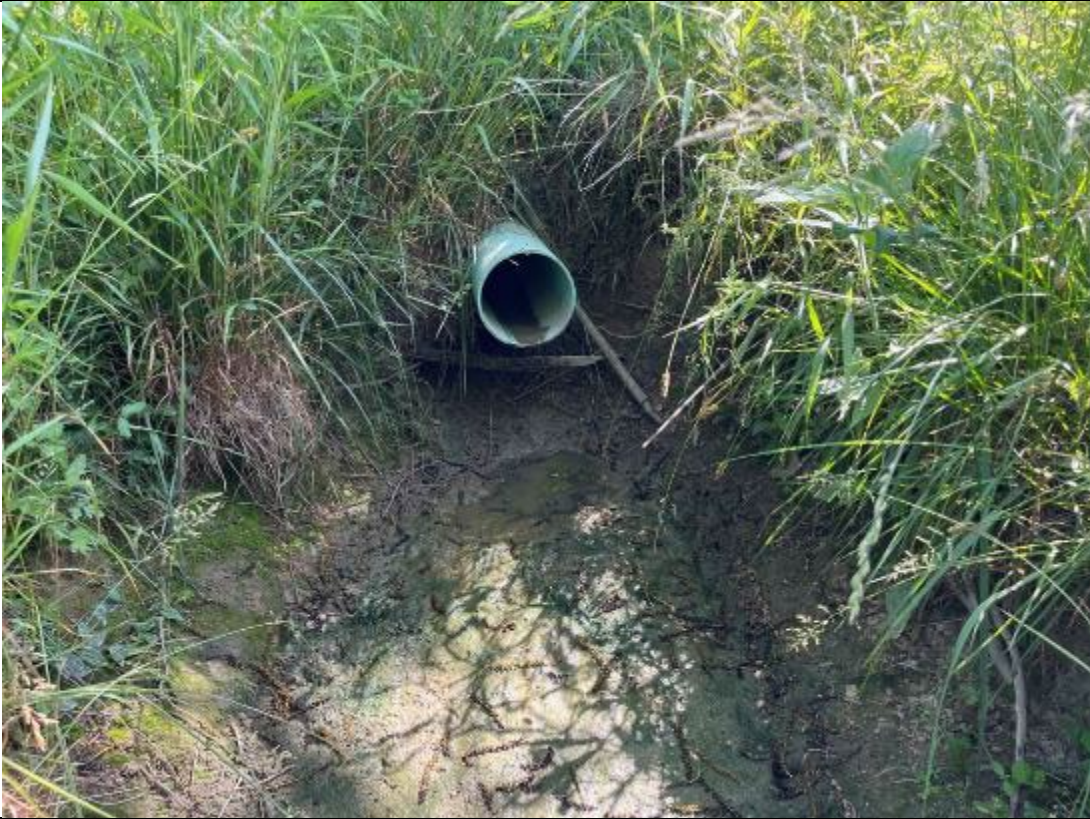
Photograph: 3 | Representative view of culverts on the Site.
