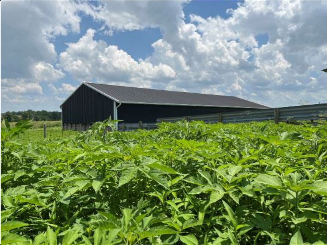
Photograph: 15 | View of the barn located on the northwestern portion of the Site.
