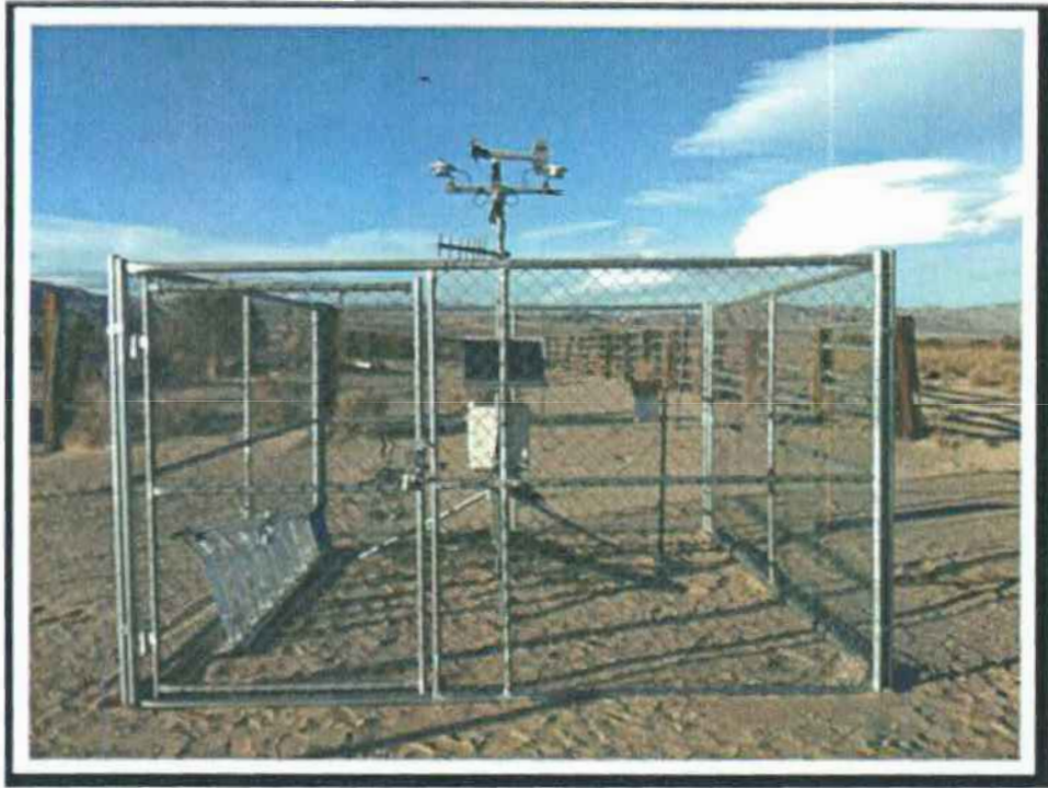
Representative Image of Meteorological Station with Enclosure
