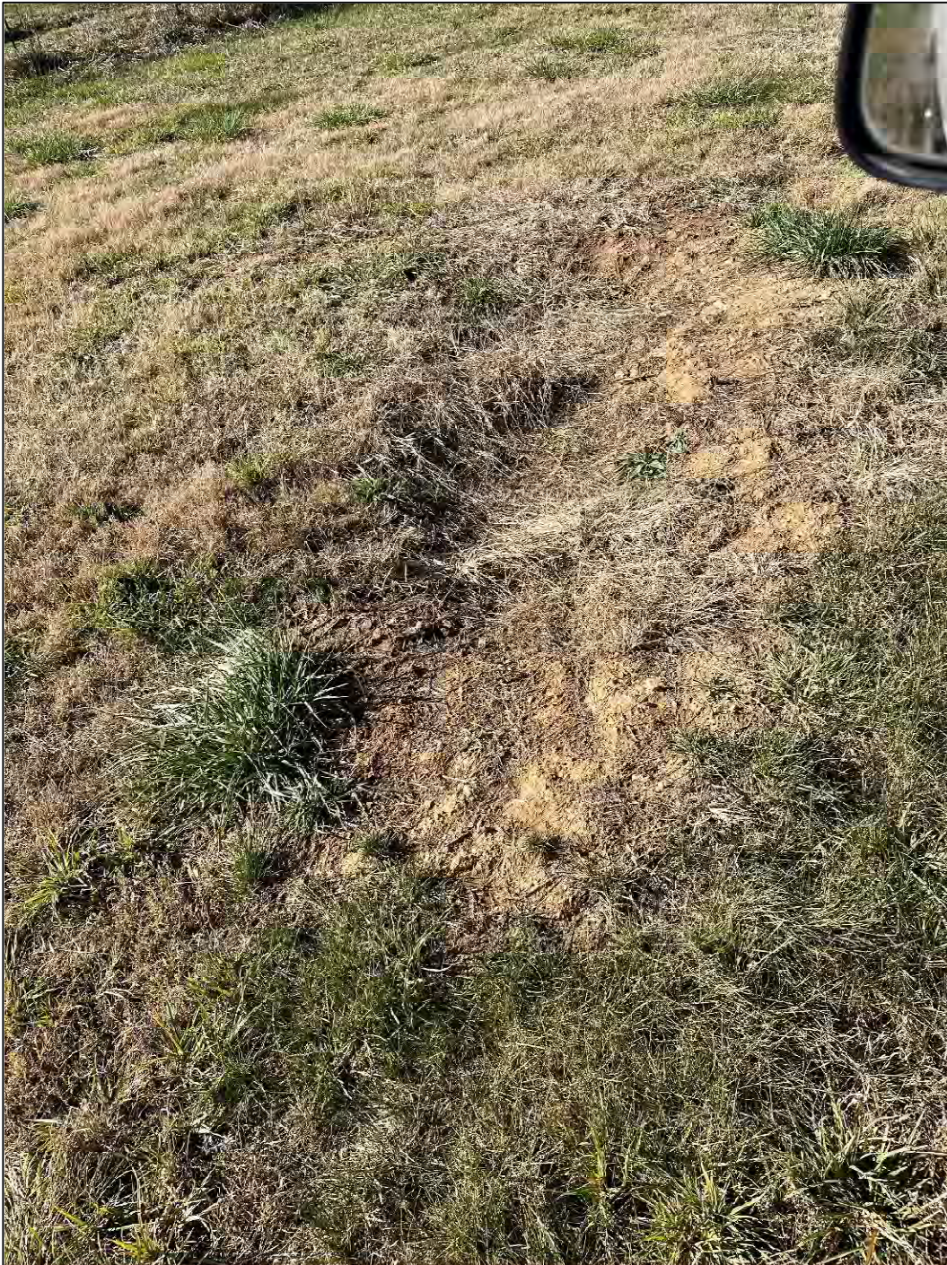
G2 observed depression 2 of 11 Approximately 265 feet South and 10 feet East from soil boring location B-13 Latitude: 37.653147 N Longitude: 85.272326 W
