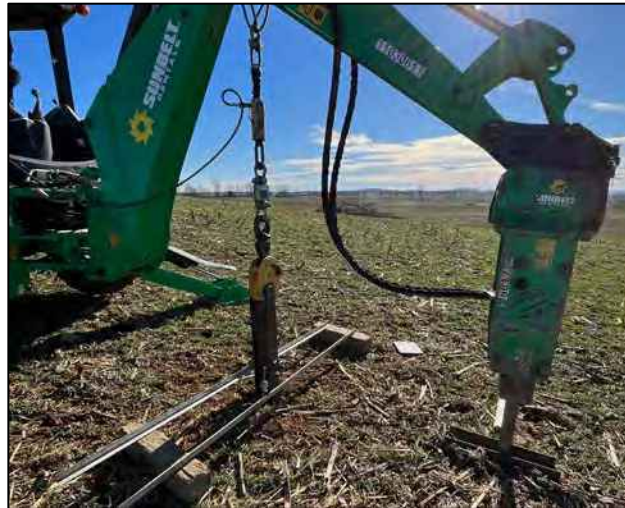
Tension Load Test Setup
