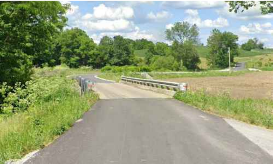
Booker Road bridge over Cartwright Creek
