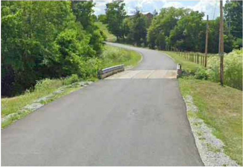
Booker Road bridge over Servant Run Creek
