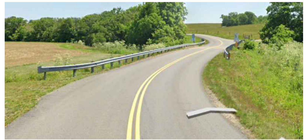
Northeast along KY 429, towards the intersection with McLain Road to the right
