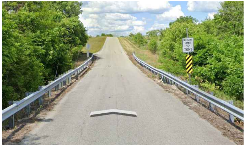
Route 3165 bridge over Servant Run Creek
