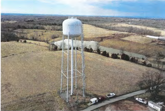
Photo shows the north side of the tank.
