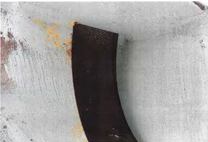
Photo shows the roof vent is equipped with a fine mesh insect screen.
