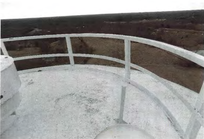
Photo shows the topcoat along the south section of the roof has lost its gloss.
