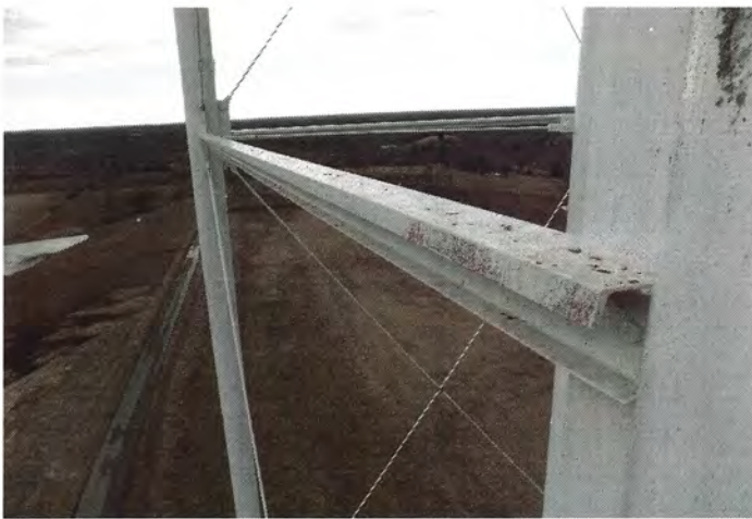
Photo shows an area of erosion where the red primer can be seen along the north facing upper strut.
