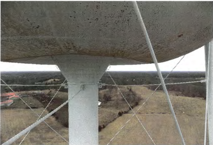
Photo shows the torus bowl and riser cone. Mildew is present but no rust was noted.
