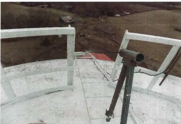
Photo shows the upper bracket of the cable style climber safety device.
