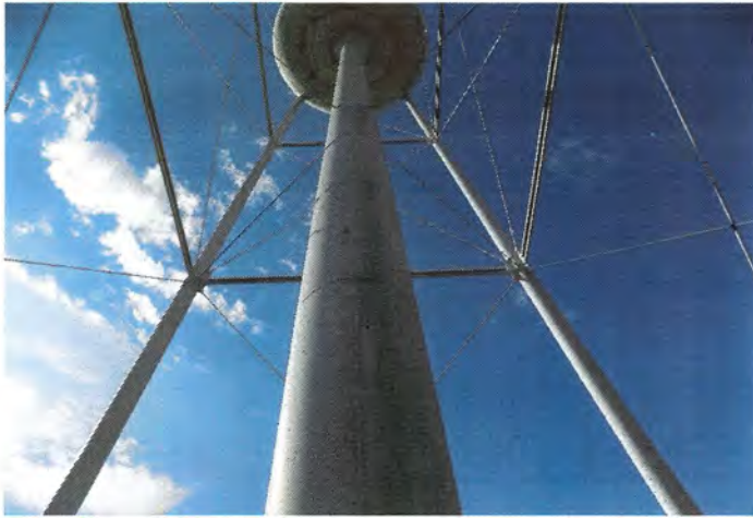
Photo shows an overall view of the riser. Minor mildew is present.
