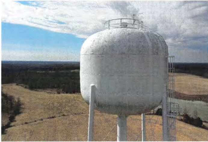
Photo shows minor mildew present along the north section of the shell.
