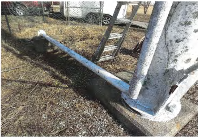
Photo shows the lower section of the 4" diameter overflow pipe.
