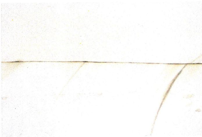
Photo shows the west section of the roof finger panels and upper knuckle. Rust bleed is present along the welded and lapped seams.
