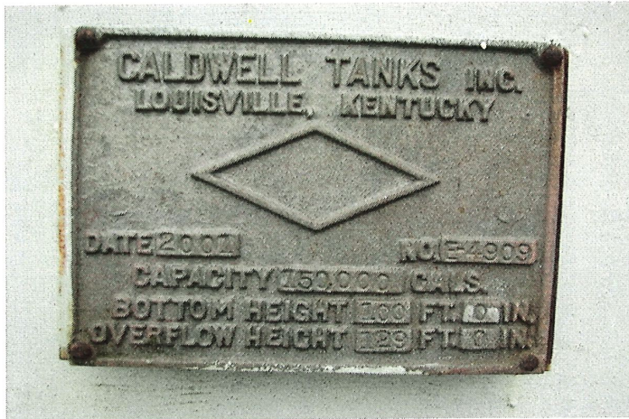
Photo shows the tank nameplate. The tank was constructed by Caldwell Tanks in 2001.
