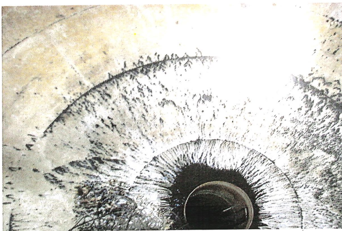
Photo shows an overall view of the bowl prior to cleaning.
