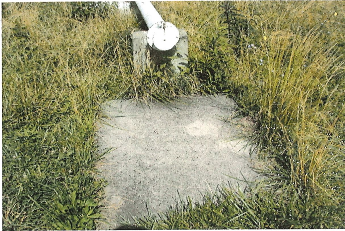
Photo shows the 6' X 4' concrete overflow splash pad.
