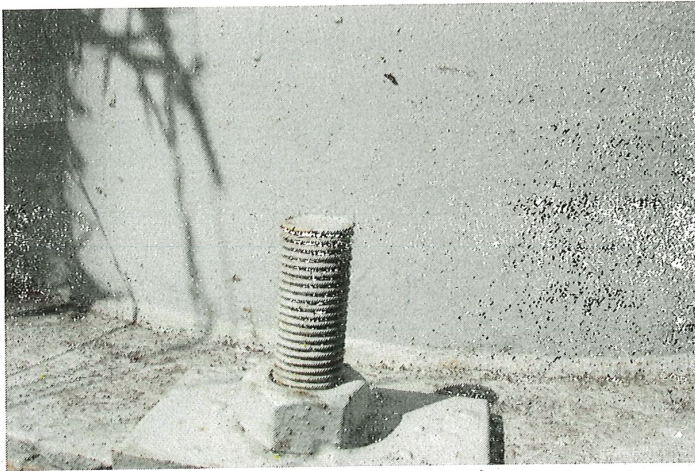
Photo shows one of four 1" diameter riser anchor bolts.
