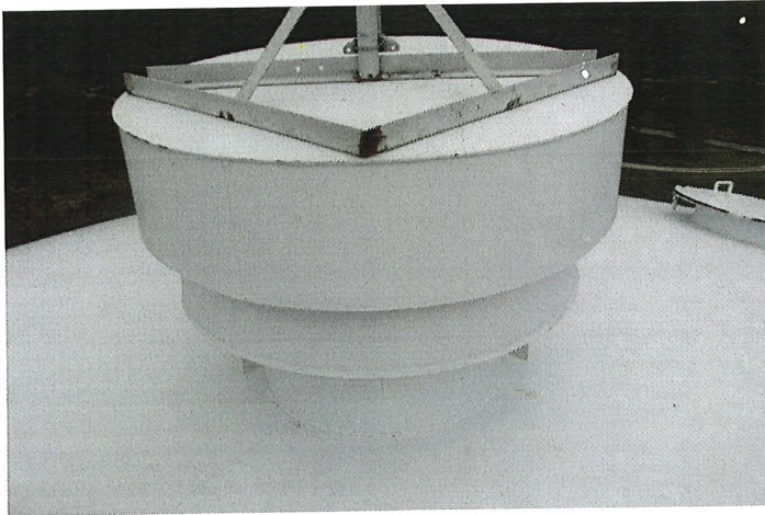
Photo shows the 24" roof vent and steel cover.
