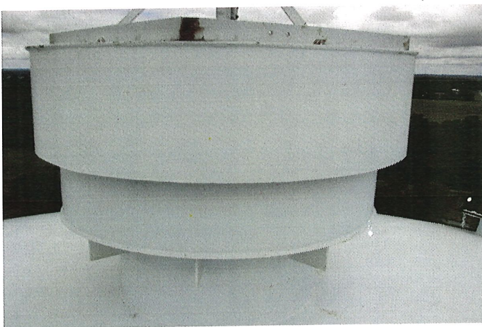
Photo shows the 42" steel vent cover and 24" roof vent neck.
