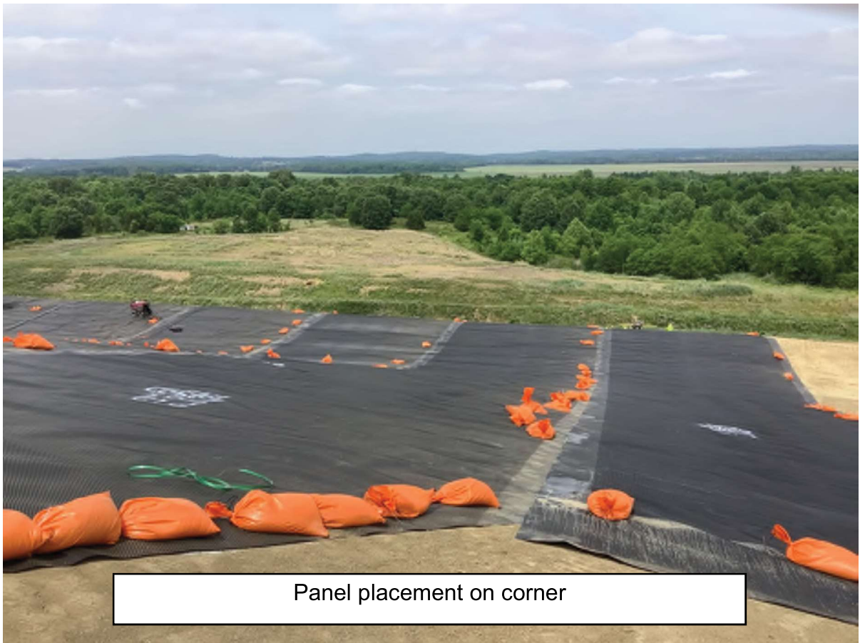
N slope prepared subgrade
