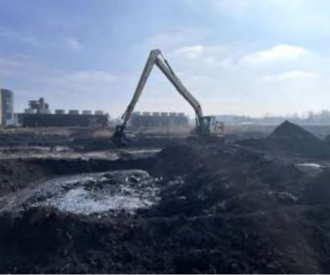
Hauling Decanted Material for Landfill Placement
