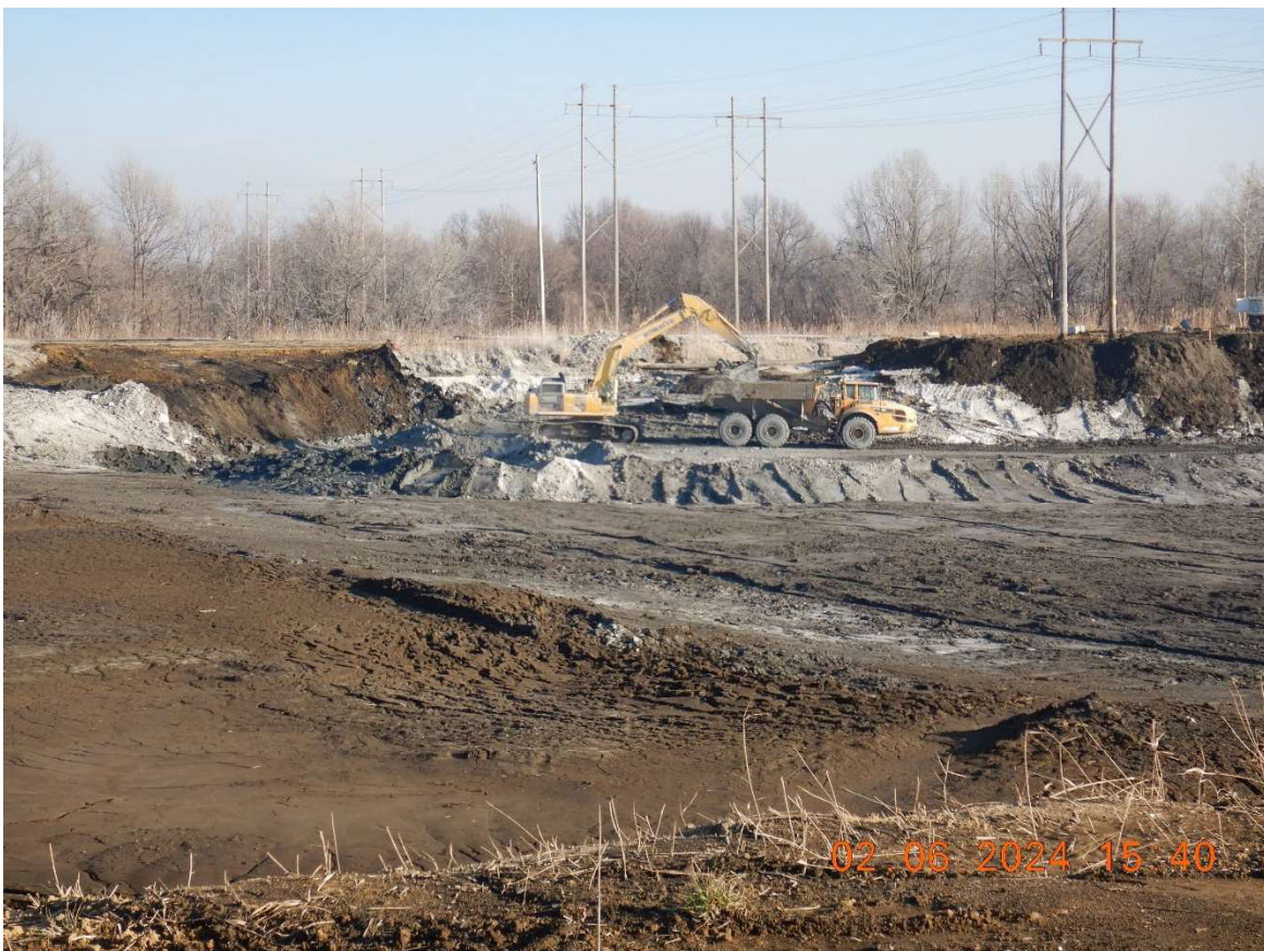
Loading trucks from loadout area to haul to placement area
