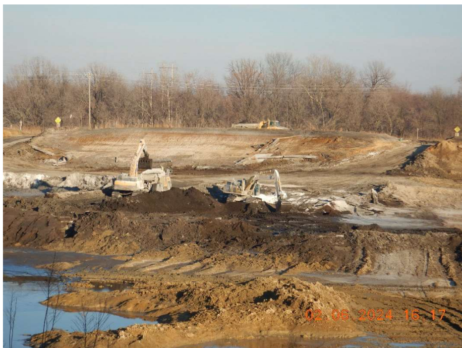
Excavating and loading CCR from southern end of ash pond
