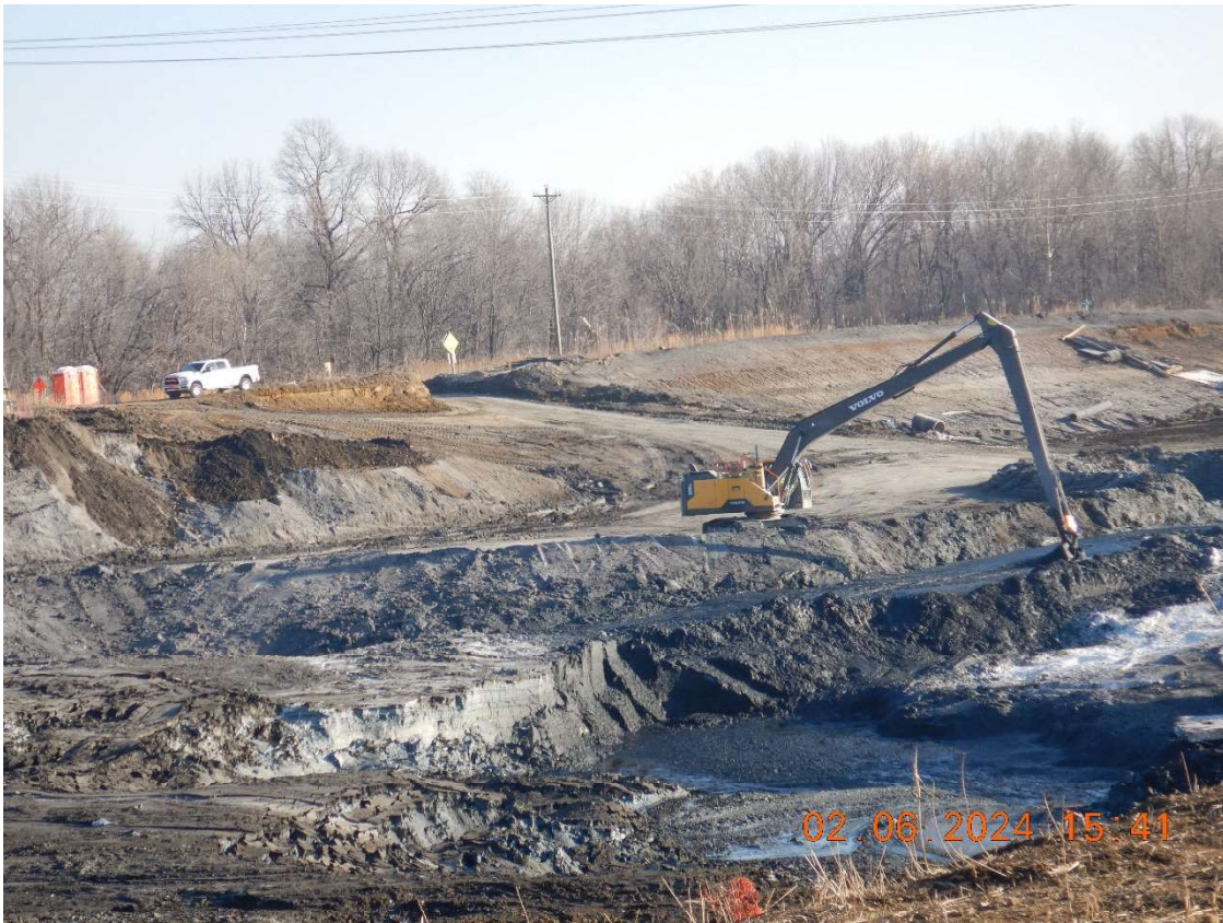
Mixing lime with wet CCR in pond mixing cells
