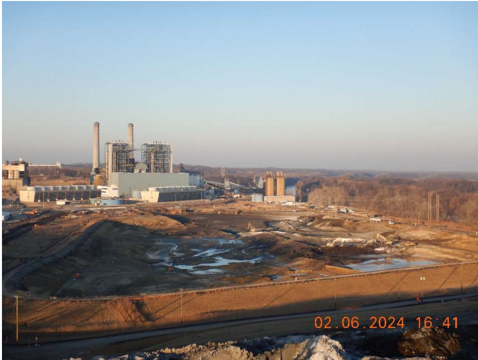
Excavating and loading CCR from southern end of ash pond
