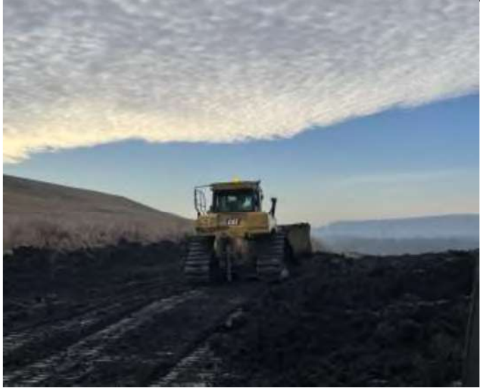
Material Placement in the Landfill
