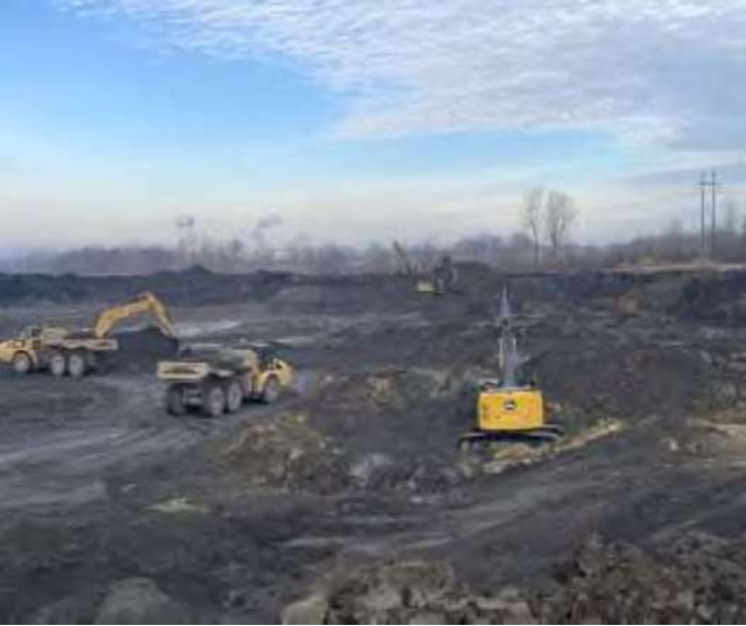
Hauling Decanted Material for Landfill Placement
