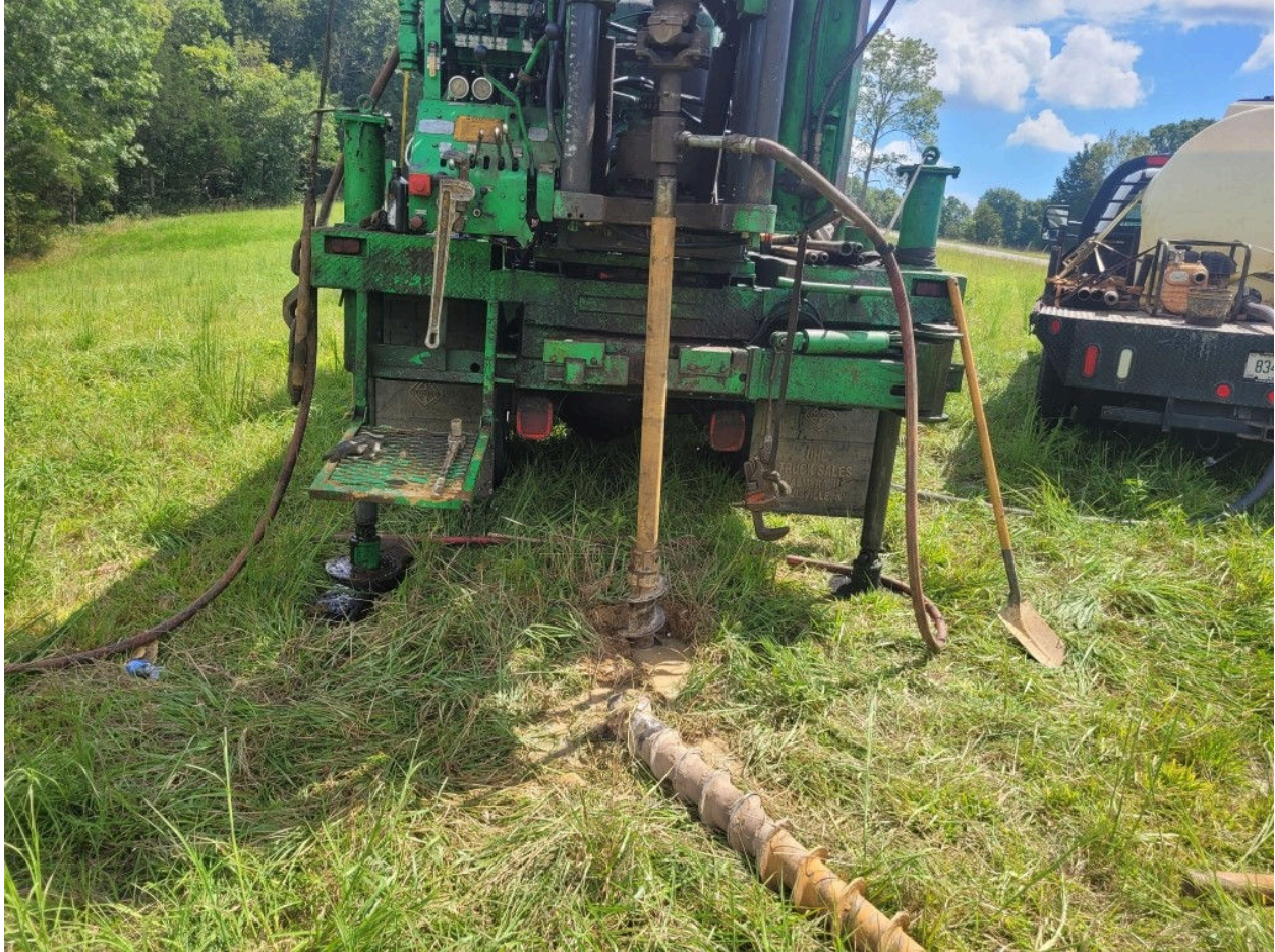
FIGURE 4: Photograph of Drill Rig and Tower Site
