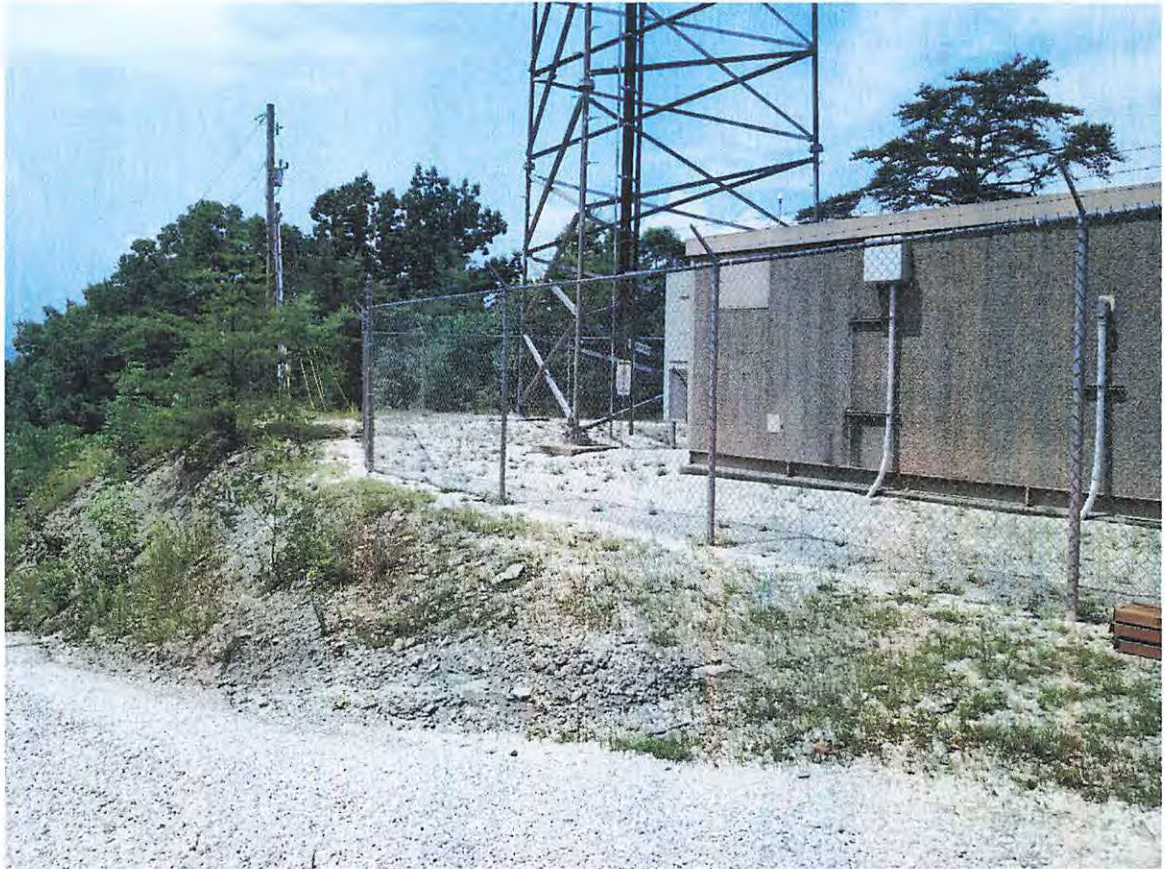
Photograph B – Existing tower site, proposed tower site to right. Note access road highwall exposing rock to be encountered during foundation construction. Photo taken from existing access road facing southwest.
