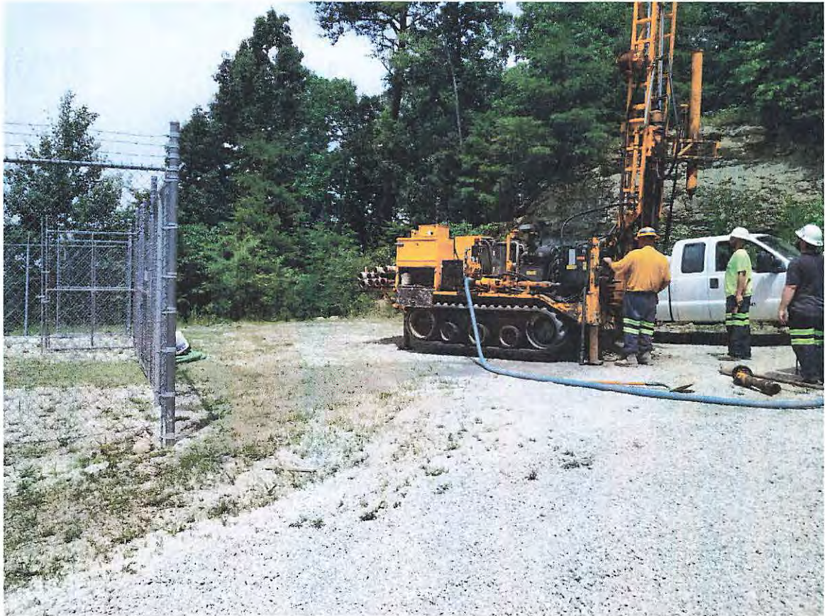
Photograph D – Proposed tower site location and approximate finished elevation. Site to be expanded beyond existing highwall in background. Drilling of corehole B-2 being conducted. Photo taken from existing access road facing northwest.
