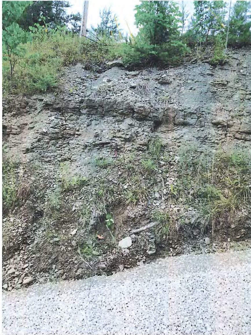
Photograph C – Access road highwall exposure showing rock to be encountered during foundation construction. Photo taken from access road facing west.
