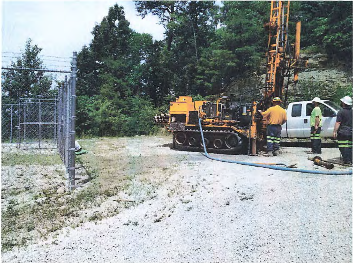
Photograph D – Proposed tower site location and approximate finished elevation. Site to be expanded beyond existing highwall in background. Drilling of corehole B-2 being conducted. Photo taken from existing access road facing northwest.
