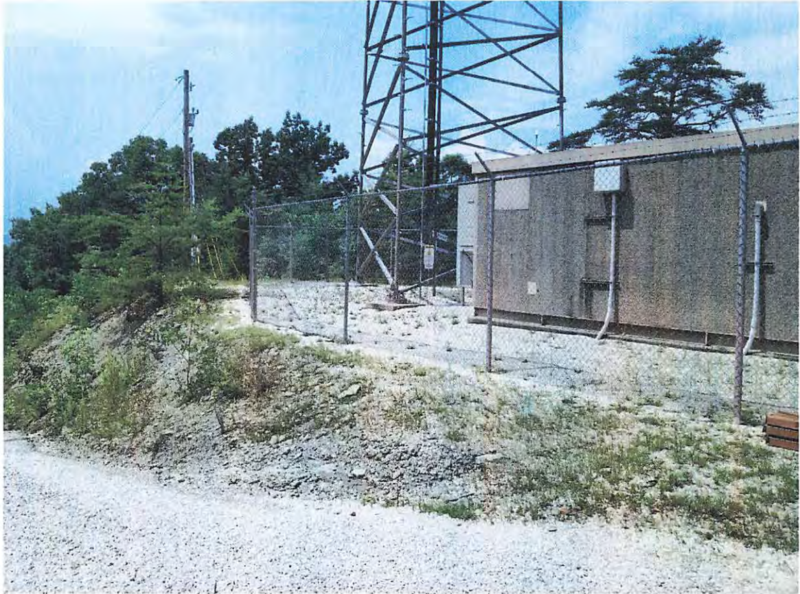
Photograph B – Existing tower site, proposed tower site to right. Note access road highwall exposing rock to be encountered during foundation construction. Photo taken from existing access road facing southwest.
