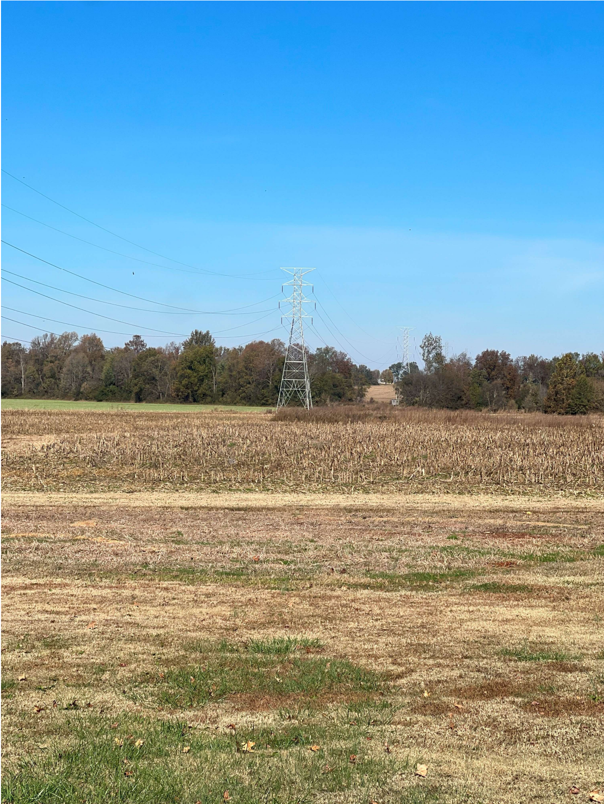
Picture (18) Stop #3 (Transmission line project will connect to, also location of project substation)
