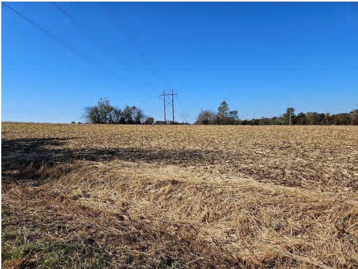
Figure C-8. Southwestern View of Future Substation Area and Existing Transmission Line
