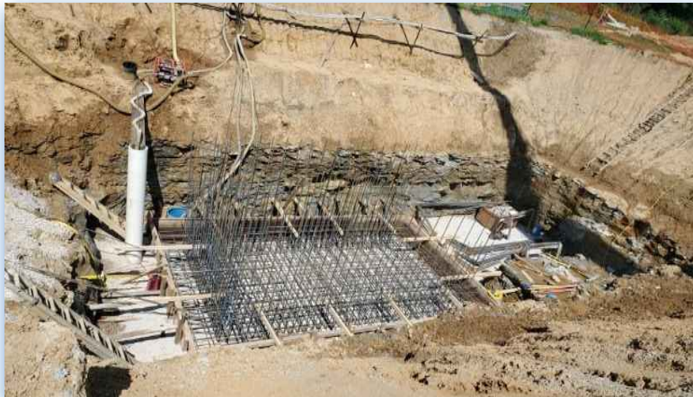
City Springs WTP New Intake. Getting ready for first concrete pour.
