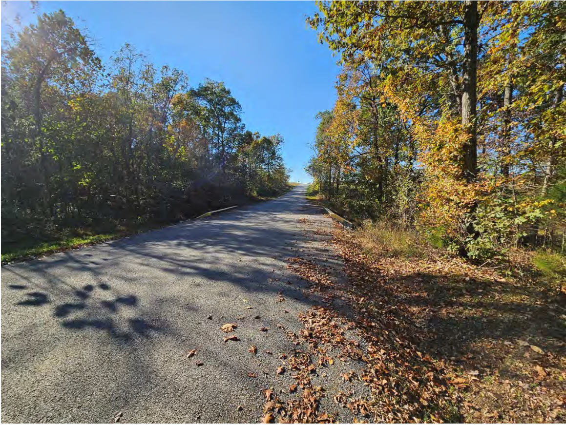
Figure C-23. Goode Road Stream Crossing Near Eastern End of Site
