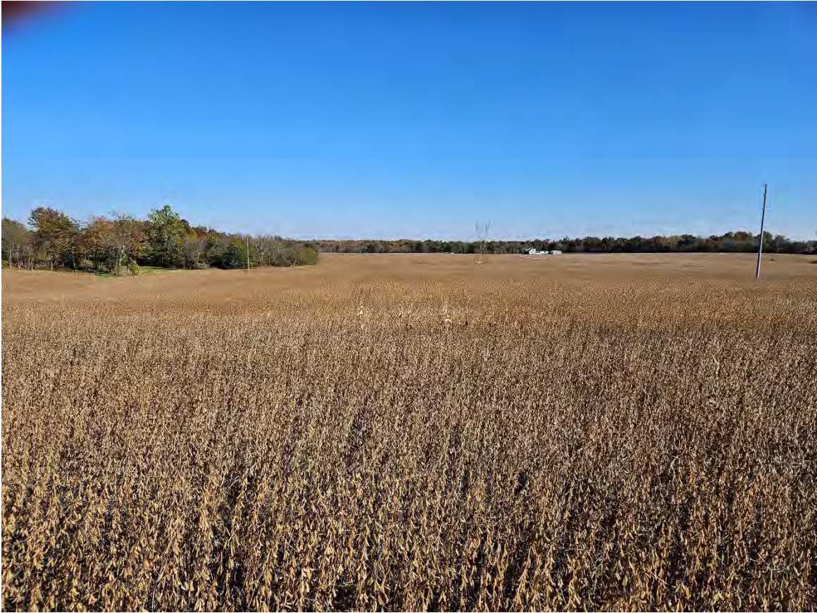
Figure C-22. View East Towards New Proposed Substation Location with Non-Participating Residence in Distance
