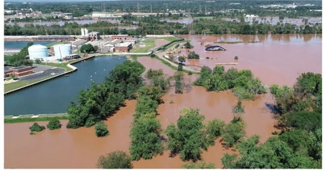
Raritan-Millstone Water Treatment Plant
