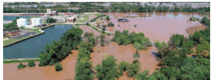
Raritan-Millstone Water Treatment Plant flood wall holds up as planned during Tropical Depression Ida, helping ensure the plant continued to provide reliable service to over 1 million customers during and after the storm.
