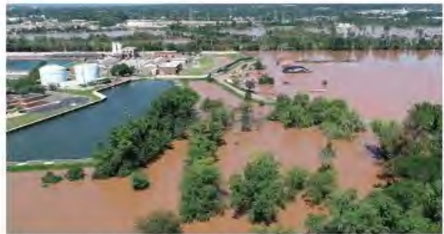
Raritan-Millstone Water Treatment Plant
