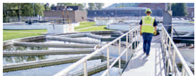
A West Virginia American Water employee monitoring operations at a treatment plant.
