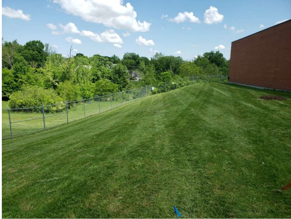
Photograph 1: The proposed project area on the west side of the existing chemical building. The area begins sloping toward the creek about 20 feet of the west wall at the north end and about 40 feet of the west wall at the south end.
