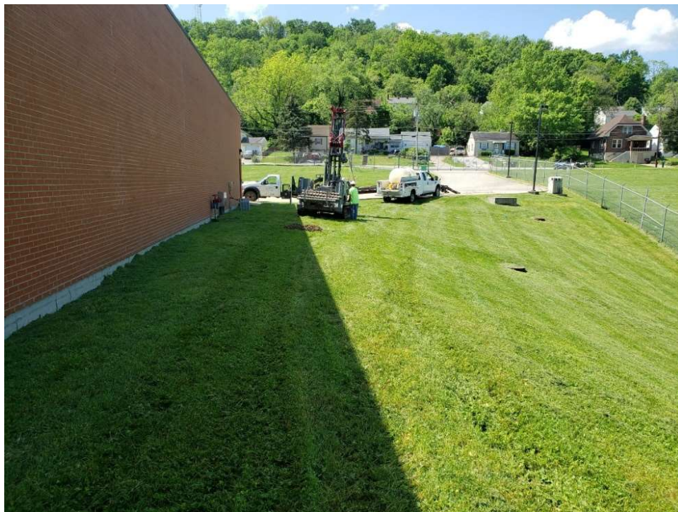
Photograph 2: The area for the generator pad is near the southwest corner of the chemical building, where the slope is more gradual and begins about 40 feet of the west wall of the chemical building
